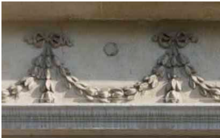
Reference: Bow motif on front elevation of 33FS.
