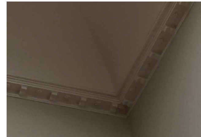
Detail of stairwell cornice, Charlotte Square, London W1
