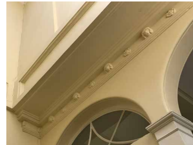
Detail of stairwell, Fitzroy Square, London W1
