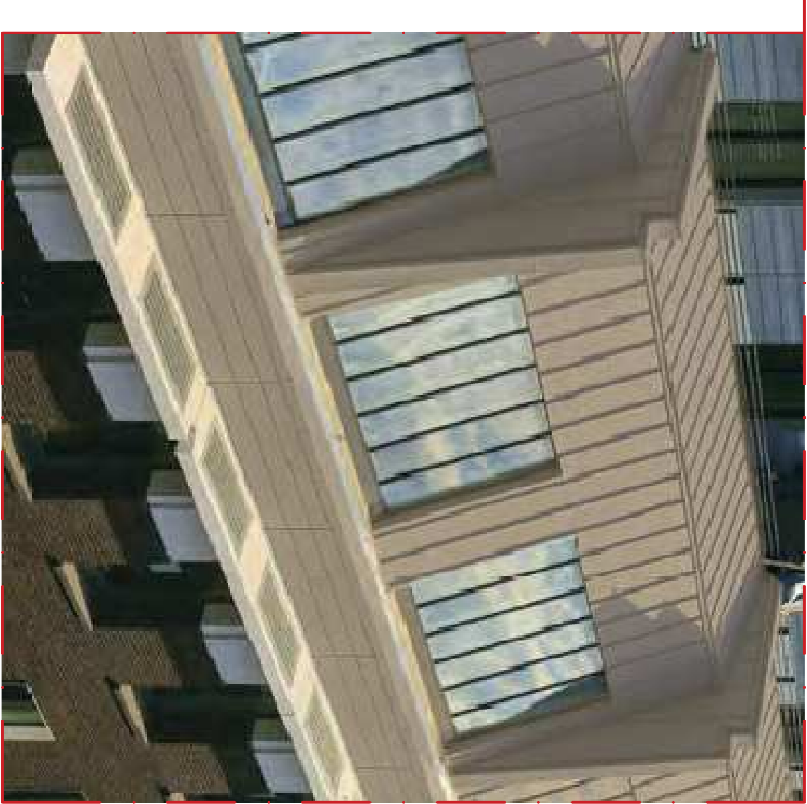
Pigmento zinc cladding to roof extension
