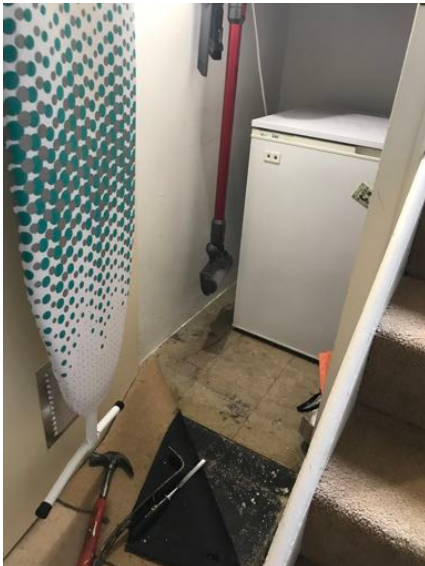
PHOTO 4. Lower Ground Floor tiles on slab.
