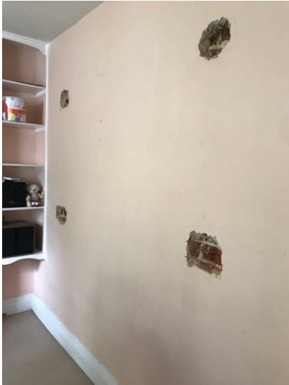
PHOTOS 7 & 8. Wall between new front and back rooms on Lower Ground Floor showing mortar removed and brickwork.
