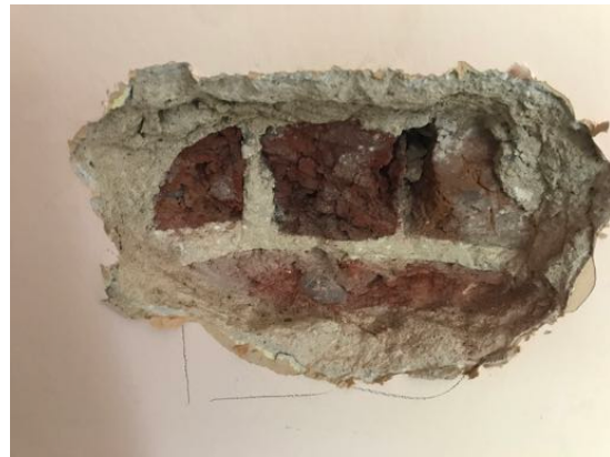
PHOTOS 7 & 8. Wall between new front and back rooms on Lower Ground Floor showing mortar removed and brickwork.
