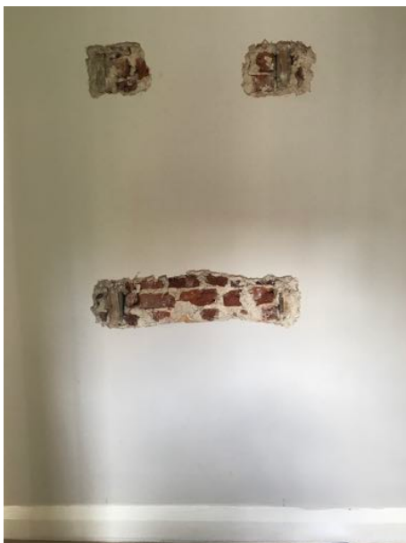
PHOTOS 2 & 3. Wall between front and back rooms on First Floor showing mortar removed, brickwork and timber posts between.
