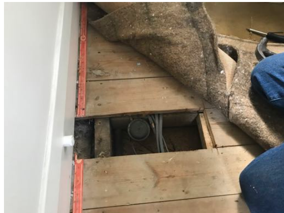
PHOTO 5. Ground Floor timber boards on joists.
