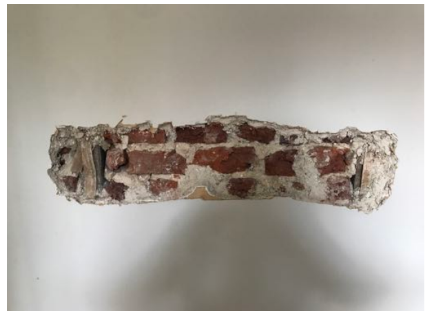
PHOTOS 2 & 3. Wall between front and back rooms on First Floor showing mortar removed, brickwork and timber posts between.
