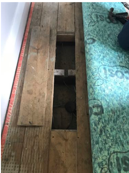
PHOTO 6. First Floor timber boards on joists.
