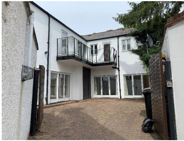
Existing building as seen from entrance gates towards courtyard
