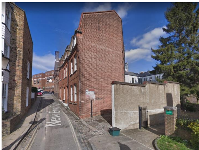
Existing building and access driveway as seen from New End Square
