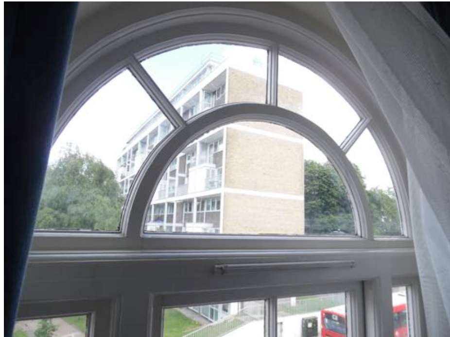
PH3 - Internal view W07
