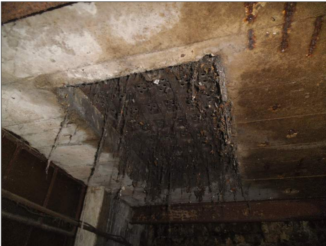
Photograph 26 – Pavement light in basement west
