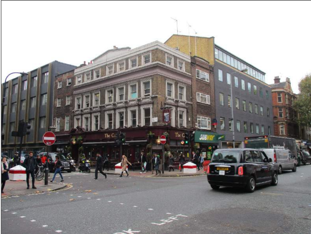
Photograph 1 – The Court, looking northwest
