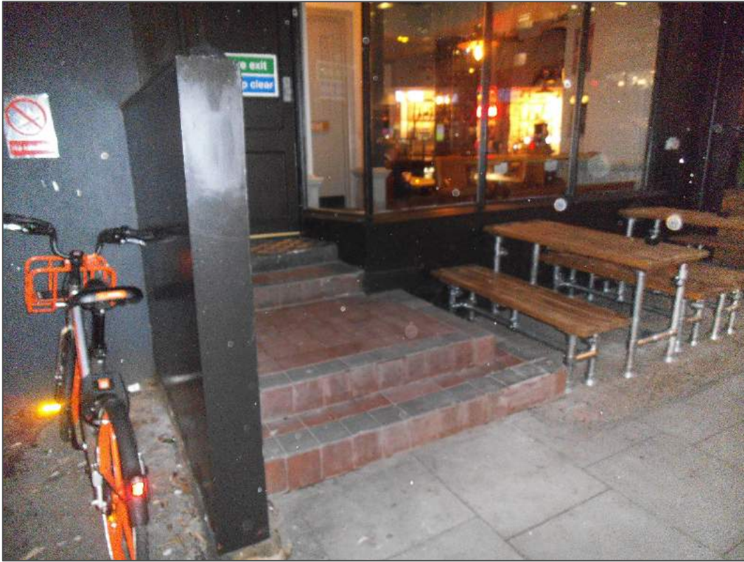
Photograph 25 – Pavement/steps over basement west
