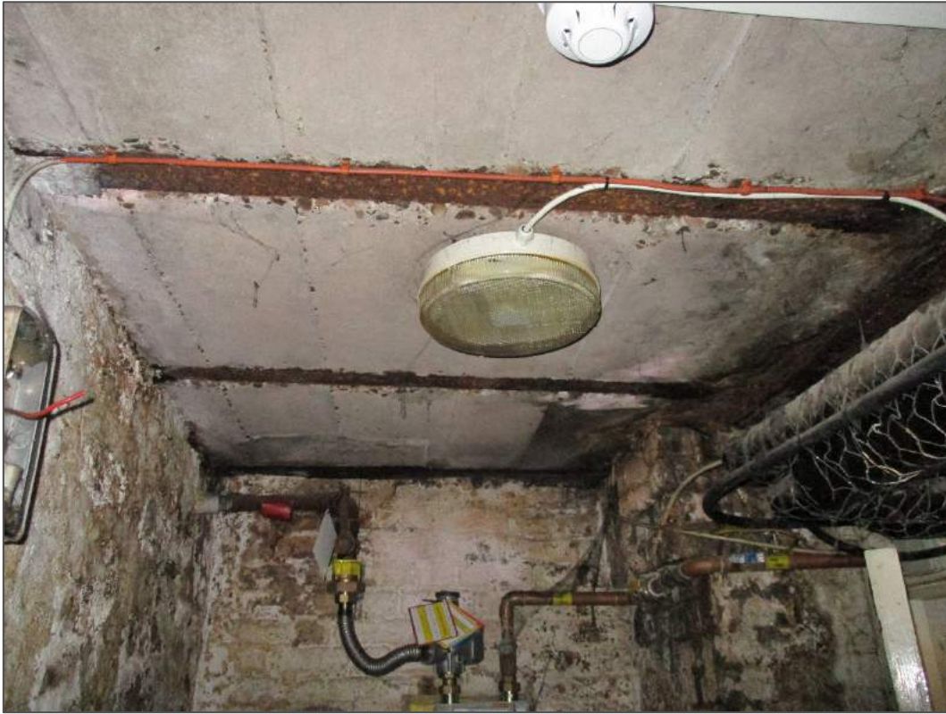
Photograph 9 – Filler joist floor in basement south
