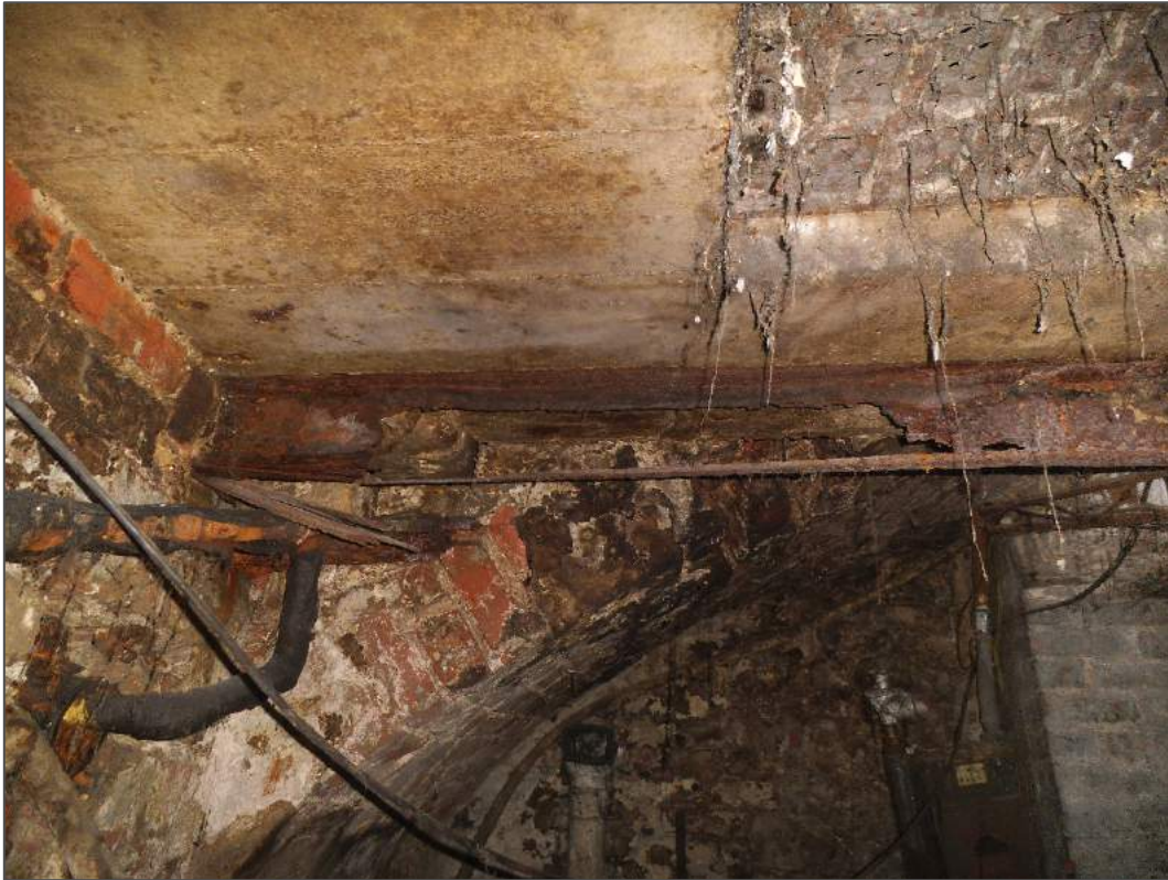
Photograph 23 – Basement west, looking west (1)
