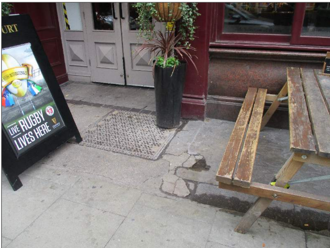
Photograph 4 – Entrance (over basement south), South elevation (2)
