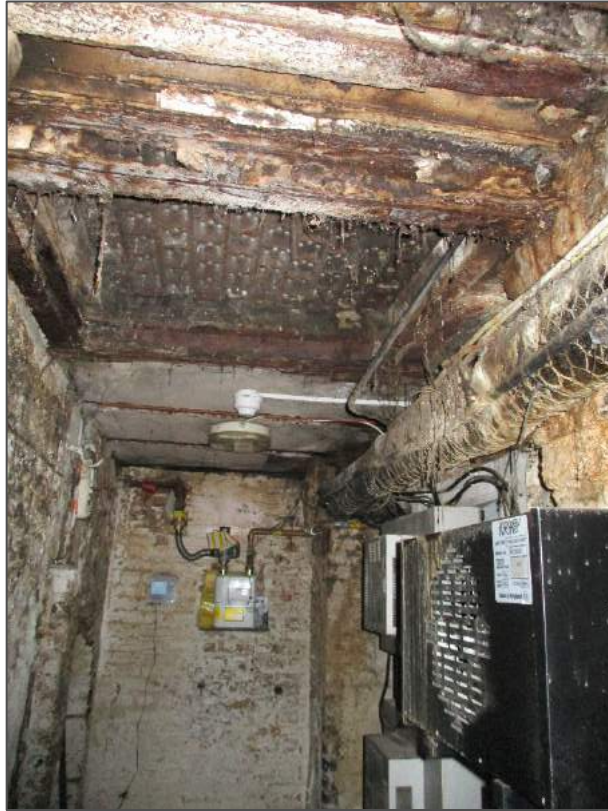
Photograph 7 – Basement south, looking west
