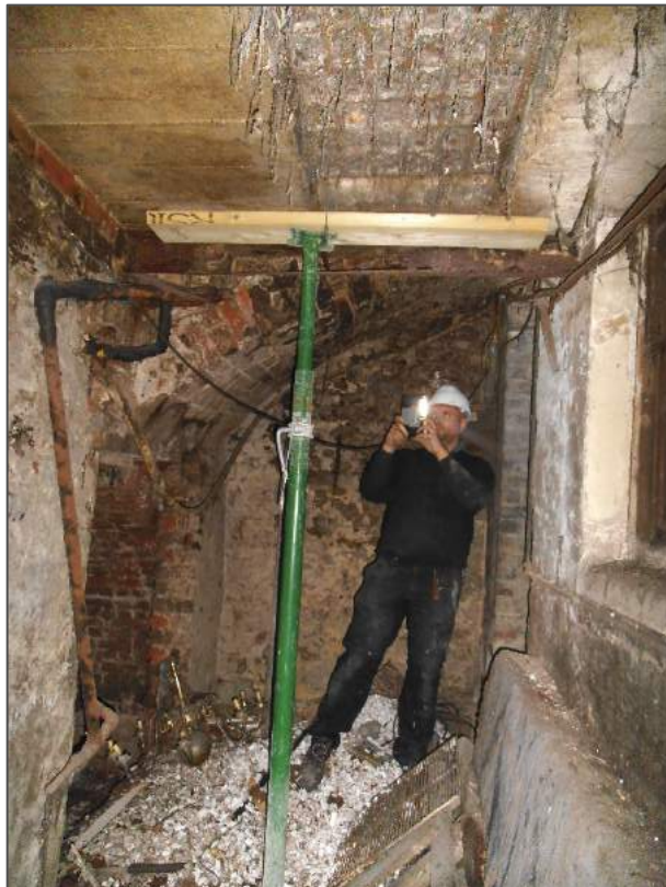
Photograph 28 – Temporary prop installed in basement west
