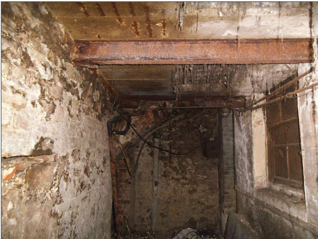
Photograph 22 – Basement west, looking west (1)
