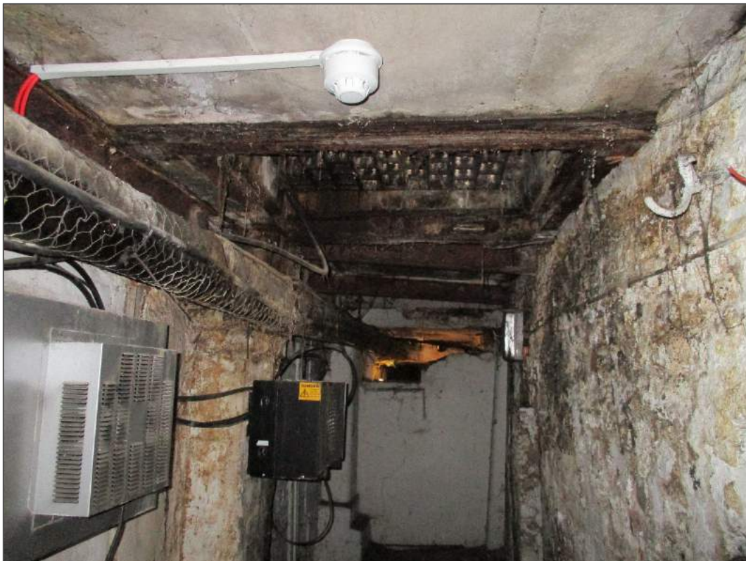
Photograph 8 – Basement south, looking east
