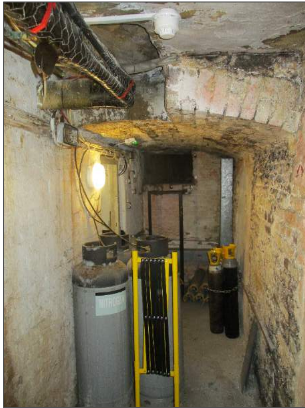
Photograph 19 – Masonry arch in basement south corridor
