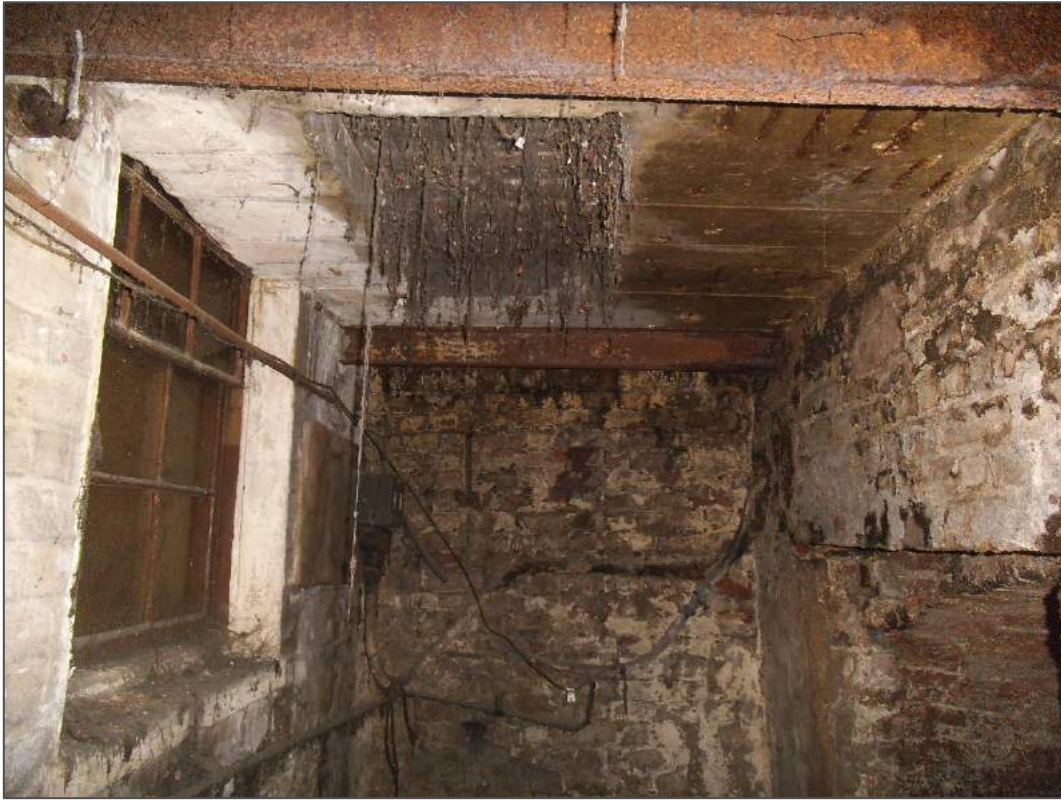
Photograph 21 – Basement west, looking east
