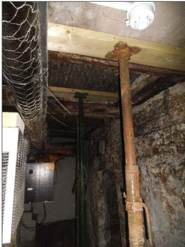
Photograph 20 – Temporary props installed in basement south
