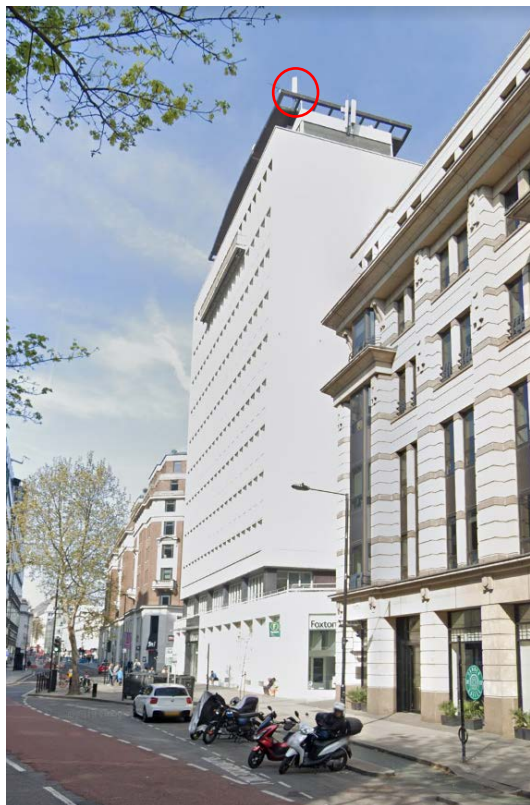
View looking West on High Holborn
