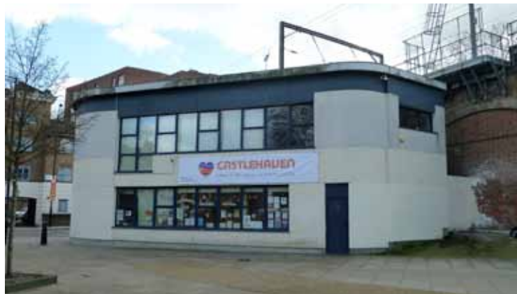
Signage on the North Elevation
