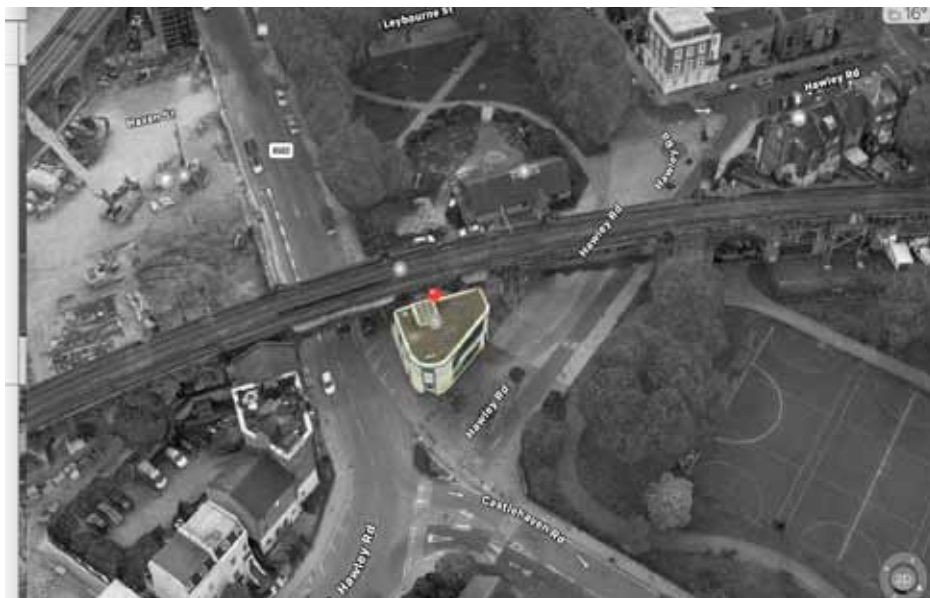
The Haven Community Centre
