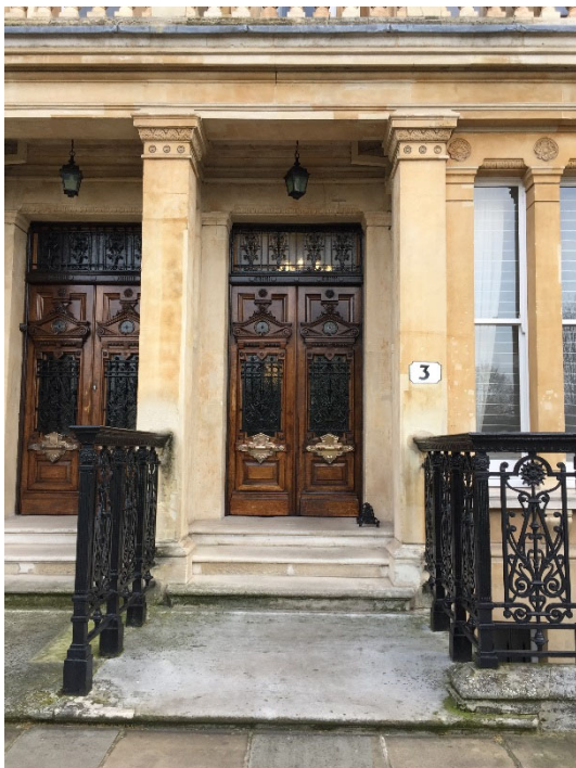
The doorway to 3 Cambridge Gate
