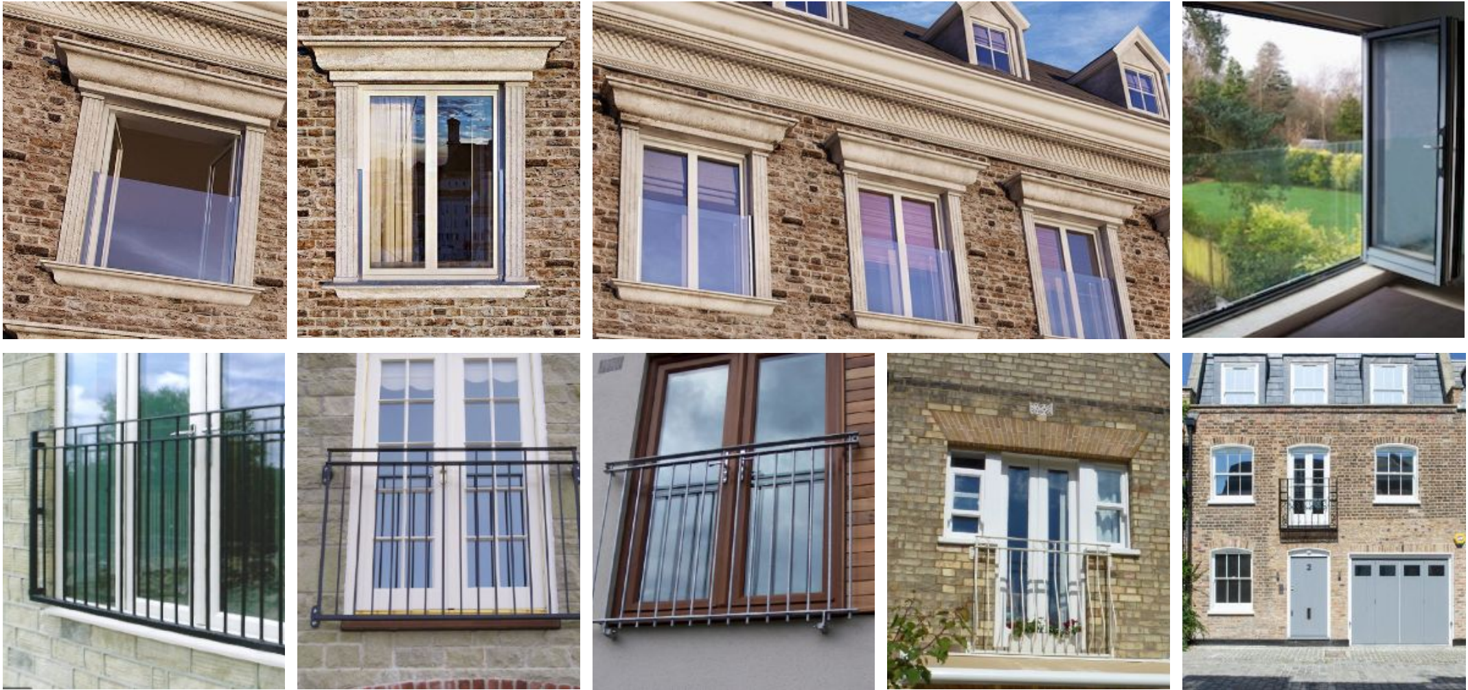
Metal railings would be an option if the glazed version was not acceptable.
