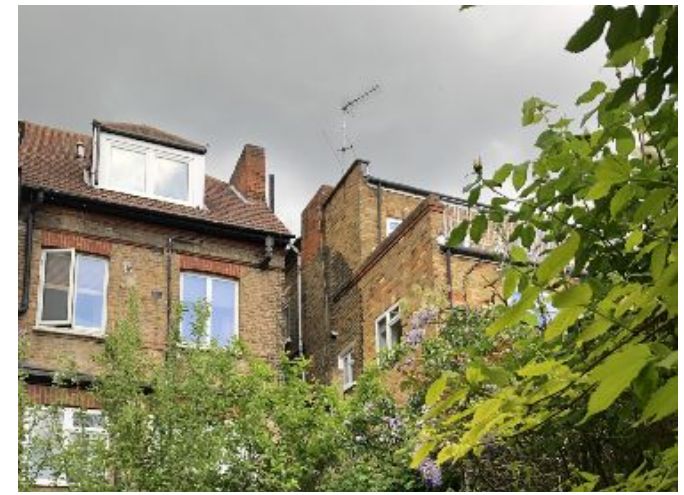
27. Existing dormer above 117 apartment
