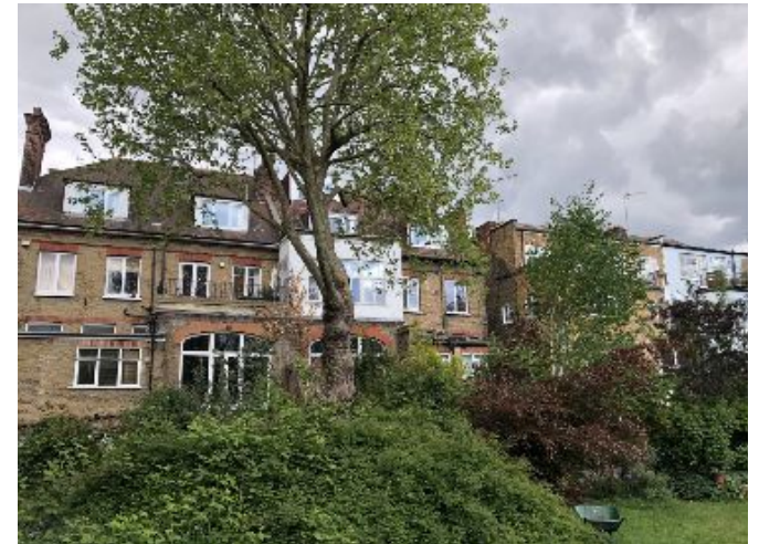
33. View of rear elevation taken further within the rear meadow.
