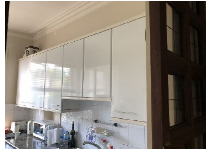
12. Wall to be opened up Kitchen side.
