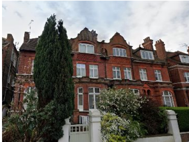
Existing Front facade of 117 Broadhurst Gardens
