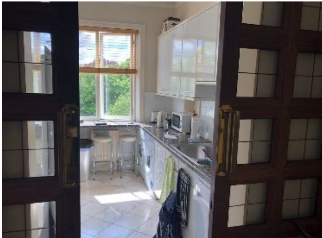
10. Kitchen to be redesigned to allow for new opening in wall (to the right).
