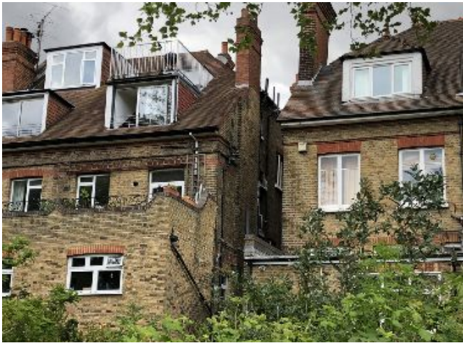
31. Views of adjacent balconies (117 to the right).
