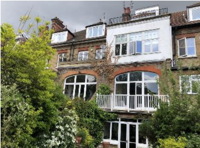
28. Further view of rear elevation.
