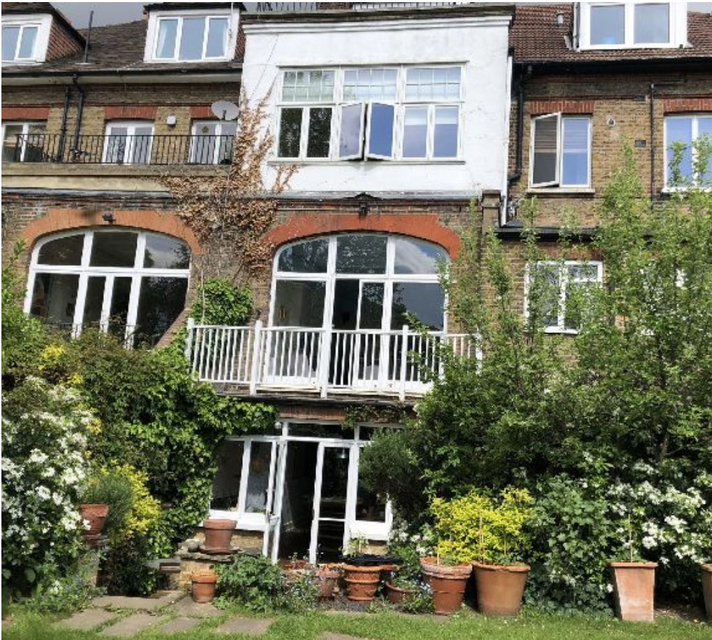
Existing Rear Elevation - White render to first floor apartment and window to be enlarged
