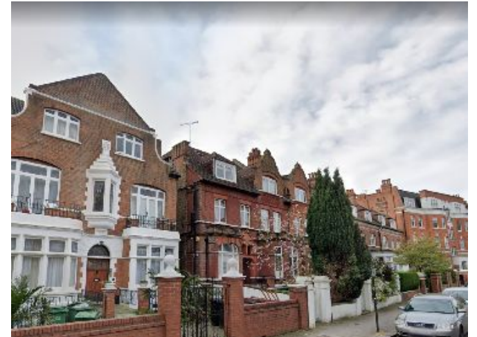
6. Existing Street view
