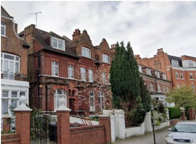
4. Street view of front facade
