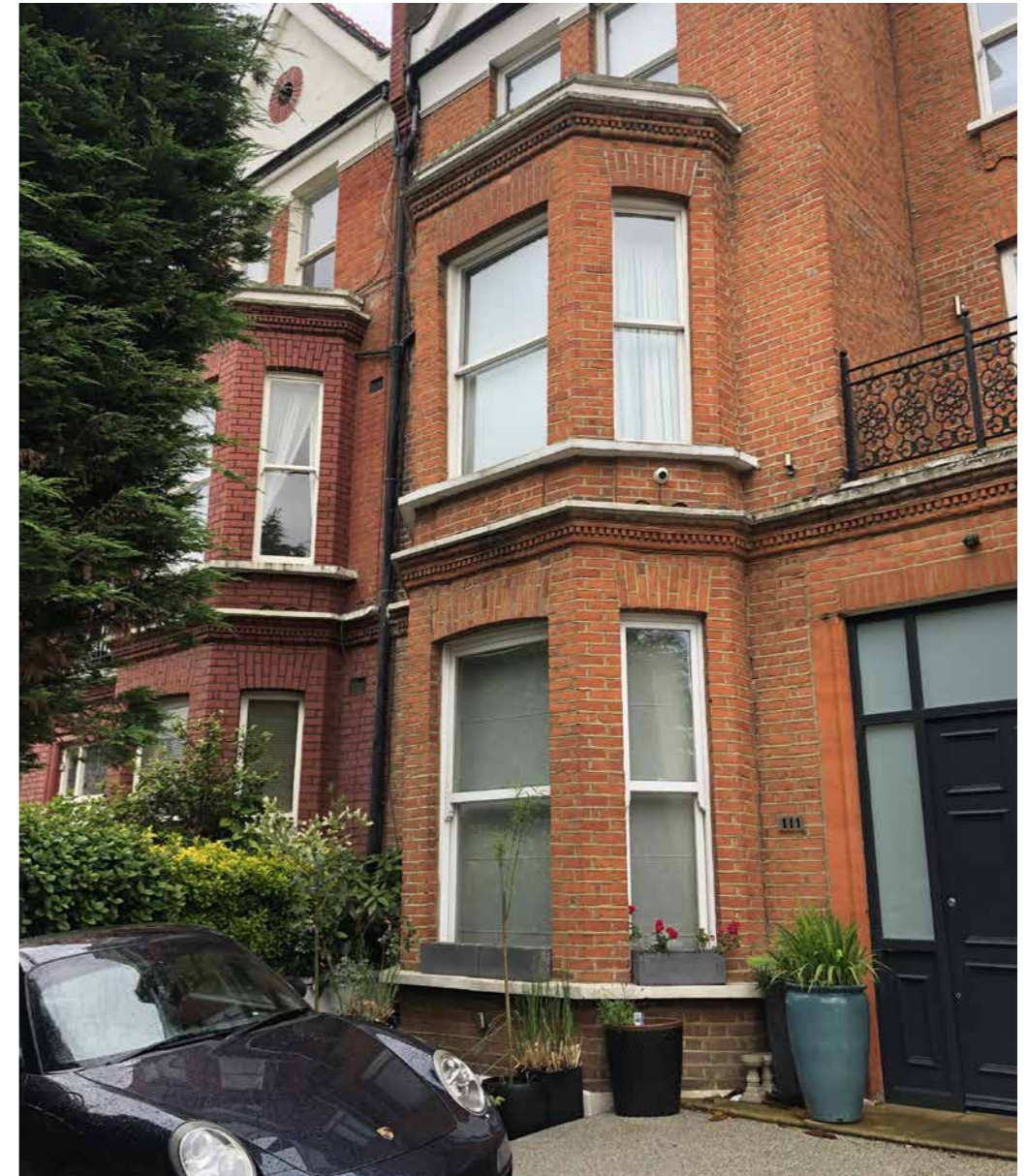
↑ Front elevation of No.111 Canfield Gardens
