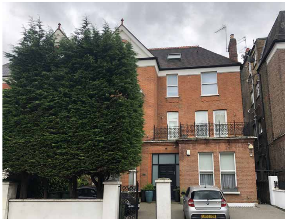
↑ Front elevation of No.111 Canfield Gardens
