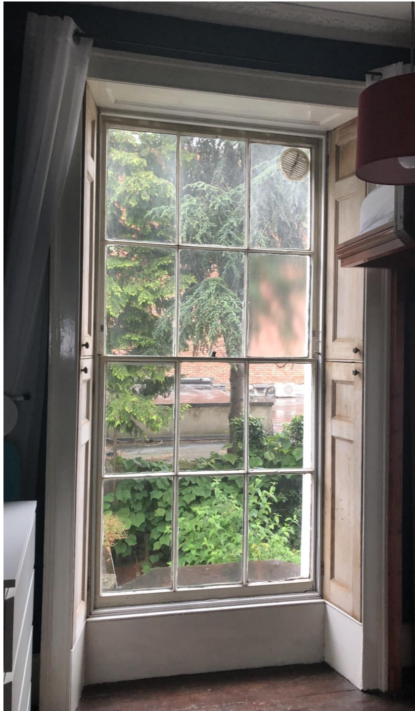
Figure 7: Internal view of window at first floor bedroom (Flat C)
