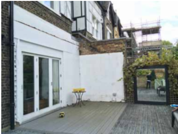
Photo 4 – Location of previous rear extension
