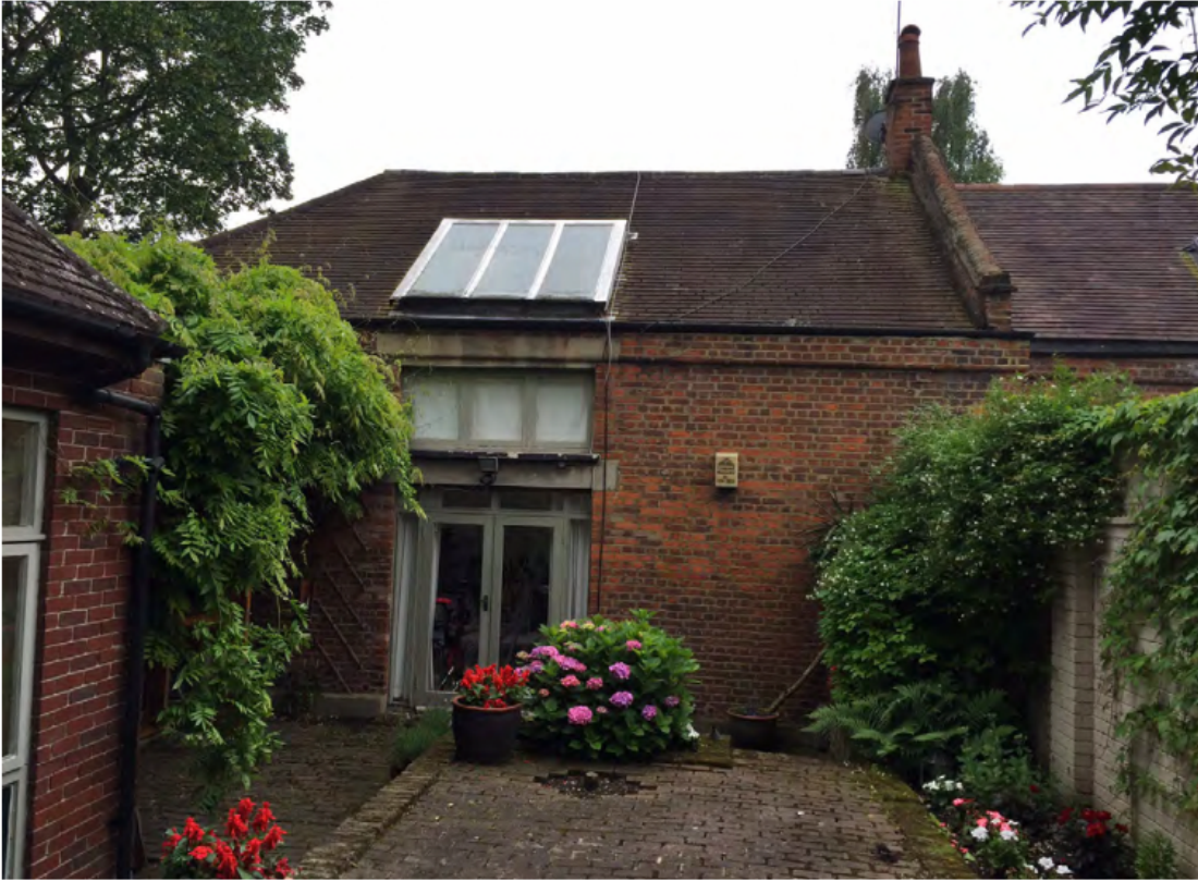
7. View of the historic studio and existing rear garden.
