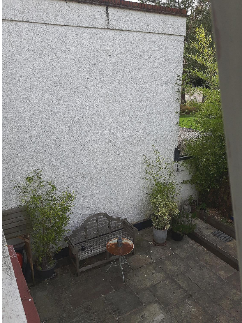
Fig. 4_ Rear elevation view from First floor rear window, on No. 1 side
