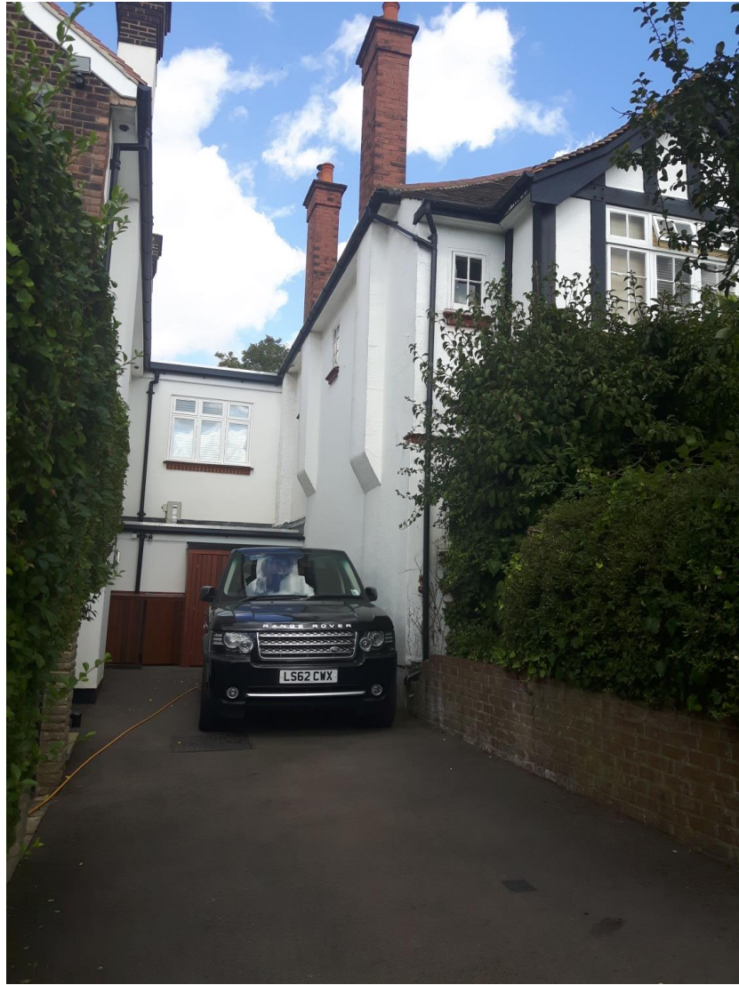
Fig. 6_ Side elevation towards No. 1 showing the side extension and garage
