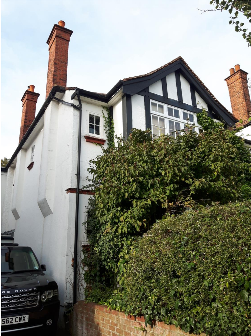
Fig. 1_ Front elevation view from the street, on No. 1 side
