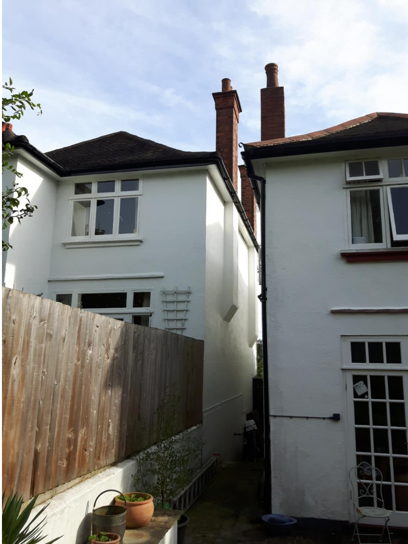
Fig. 3_Rear elevation view from the garden, on No. 5 side
