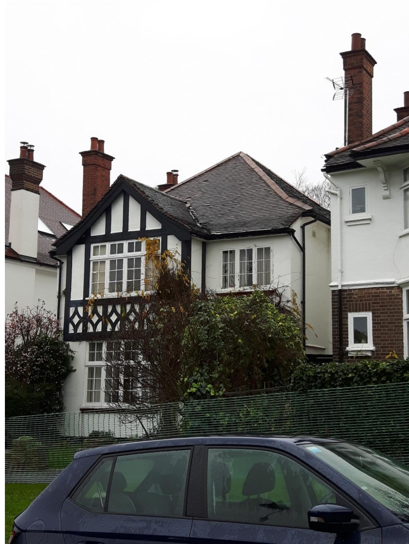
Fig. 2_ Front elevation view from the street, on No. 5 side
