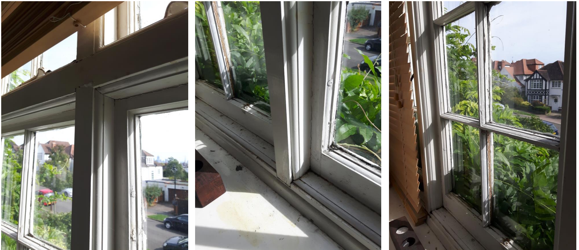
Fig.15_Details of the existing single glazed, timber casement windows.
