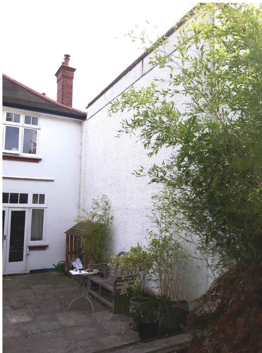
Fig 9_ Rear elevation showing the relationship with no. 1 existing two storey rear extension
