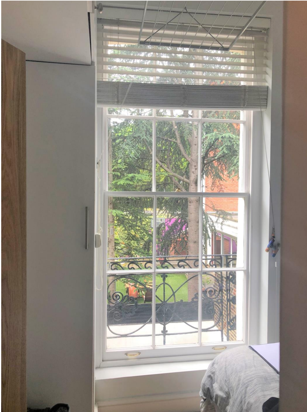
Figure 7: Internal view of window at first floor bedroom (Flat B)
