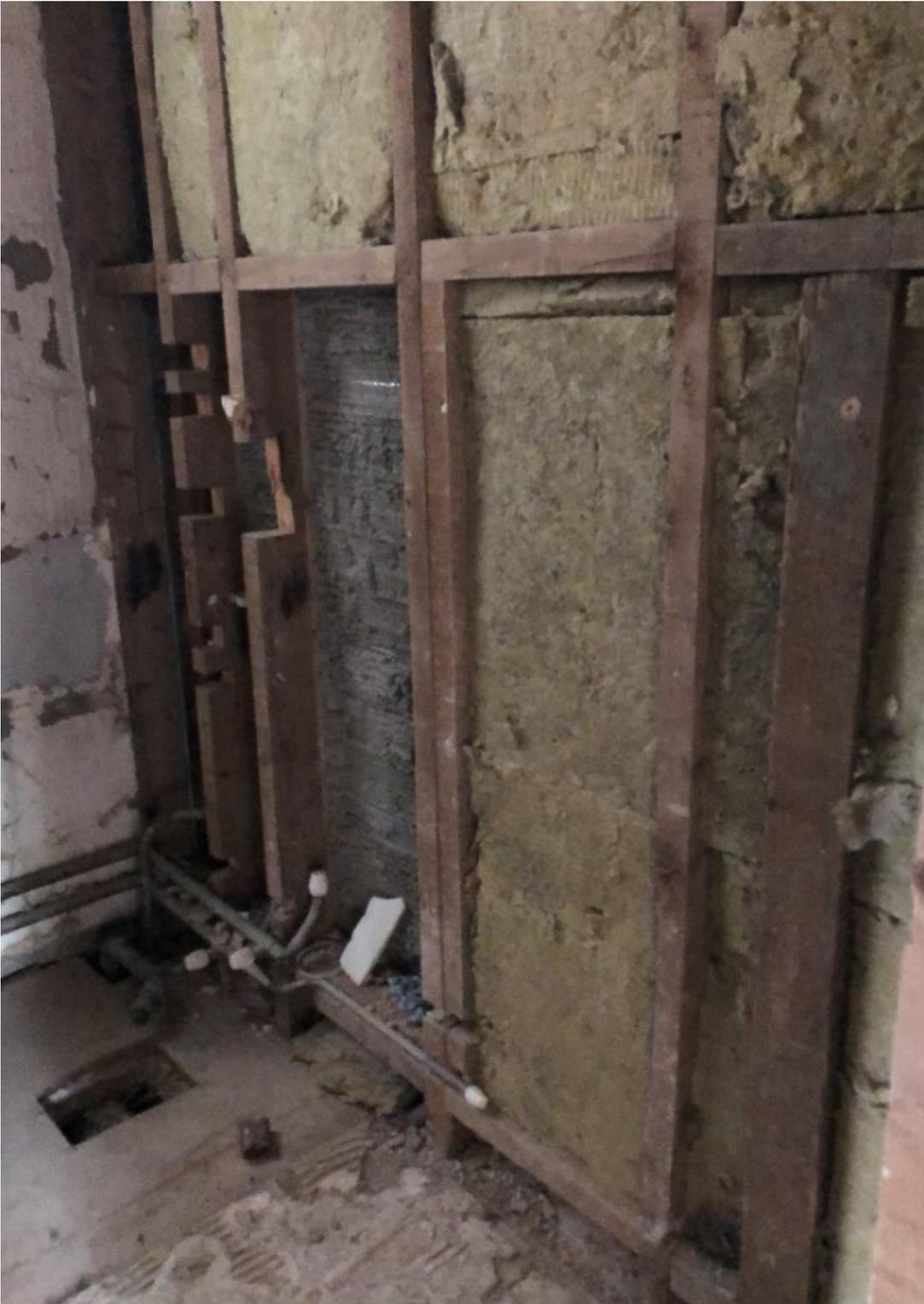
Utility Room – existing internal walls built off chipboard flooring with rockwool insulation.
