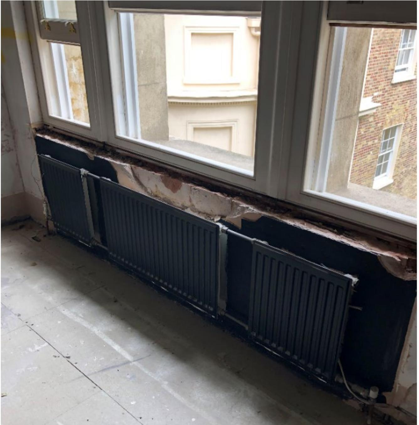
Bedroom – modern radiators remaining after removal of radiator casings (note pipes go under chipboard floor).
