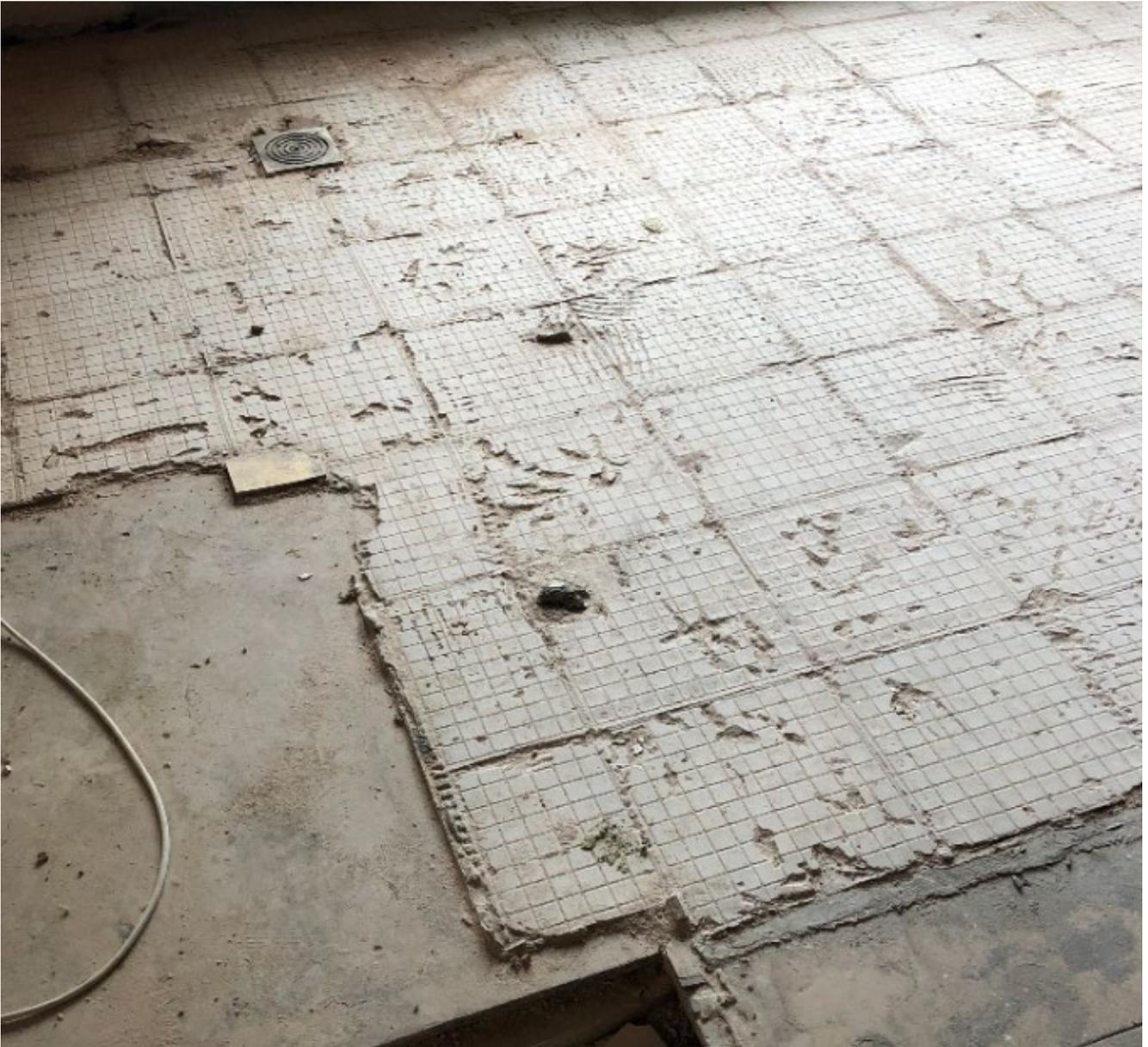
Kitchen – modern tile adhesive after removal of tiles on chipboard flooring
