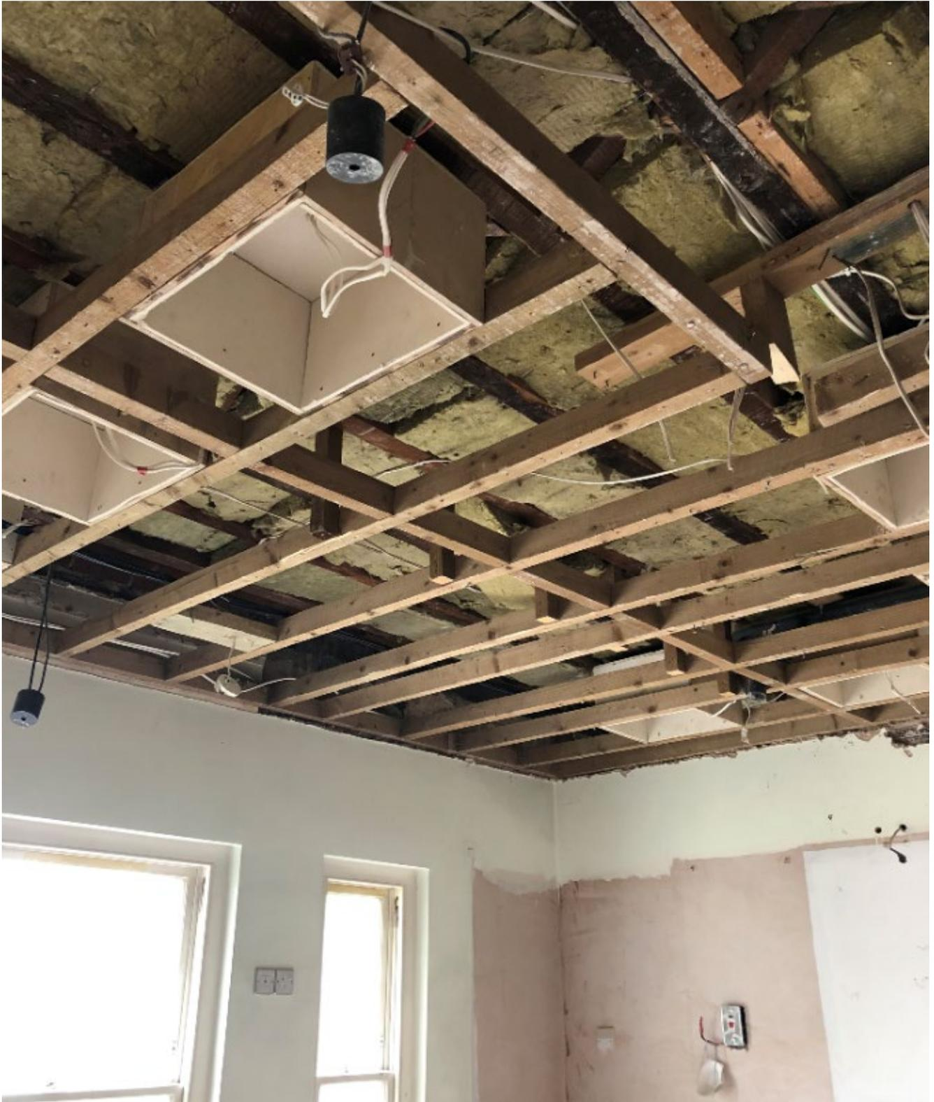
Kitchen – timber framing to ceiling showing lighting, boxes, modern wiring and insulation
