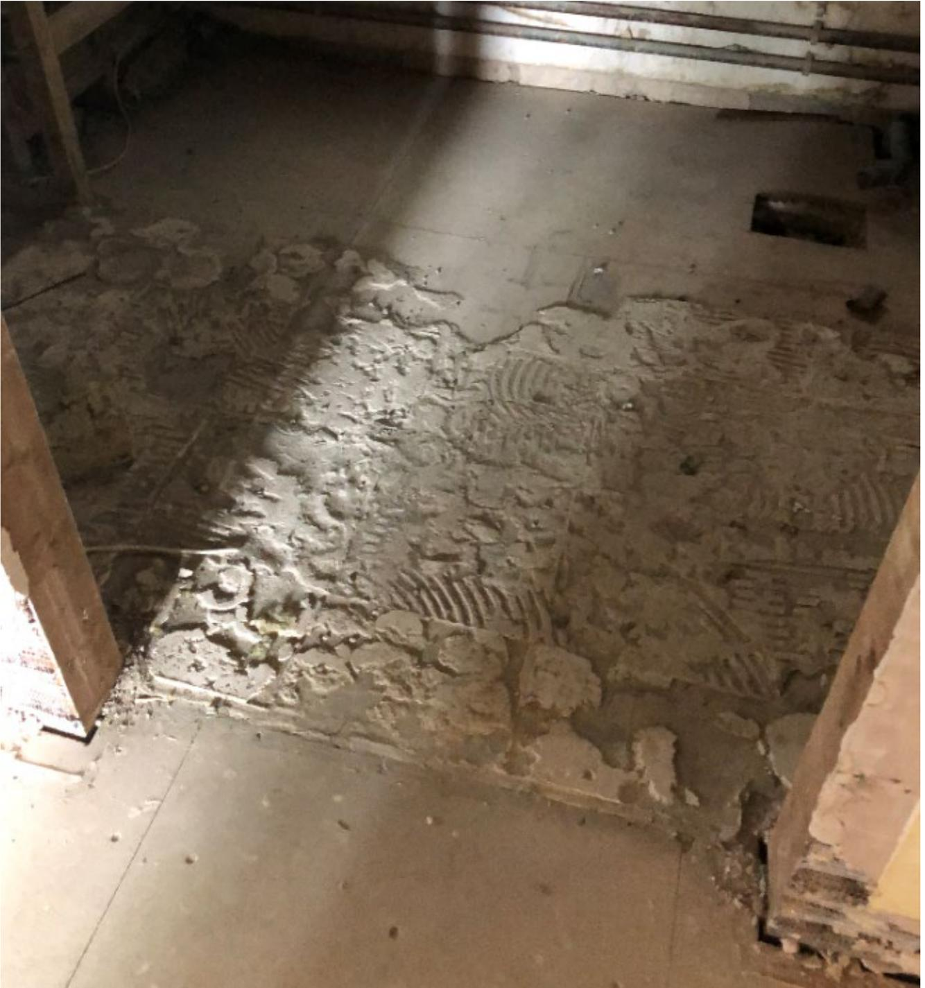
Bathroom – modern tile adhesive after removal of tiles on chipboard flooring
