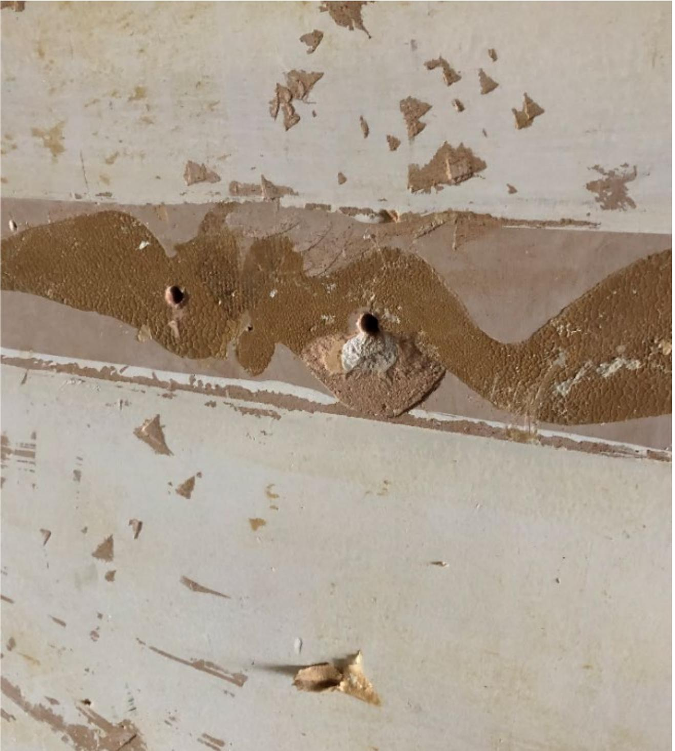
Modern Plaster to Drawing Room – showing screw holes and adhesive to removed architrave
