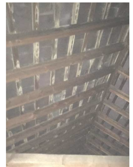
existing loft space
