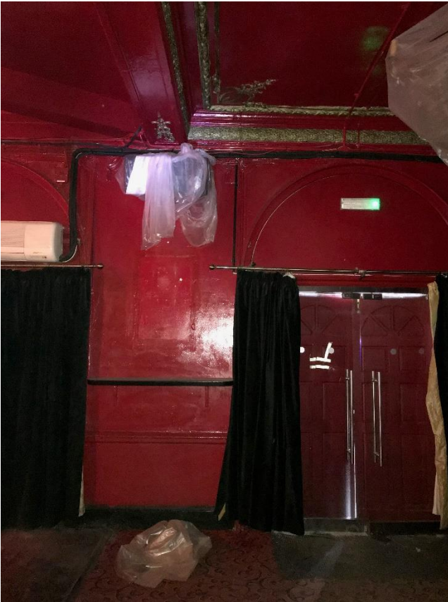
Figure 1: View of the interior of the west elevation at First floor. The proposed PFCs will be located centrally beneath the ceiling beams. The existing skirting, cornice and dado rail will be replicated on the proposed PFCs.
