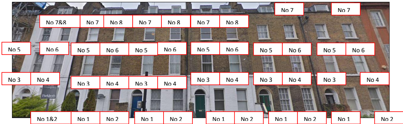
Figure 6 – No 46, No 48, No 50, No 52, No 54, No 56 and No 58 Crowdale Road
