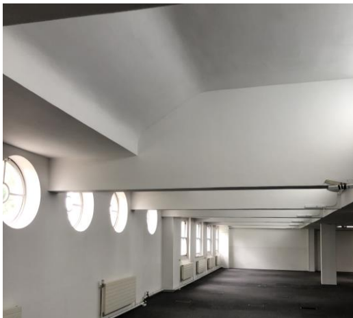
Figure 4. First floor of the former no.38 Fitzroy Square showing modern open plan layout.
