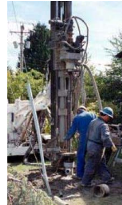
Vertical Pipe Drilling Rig
