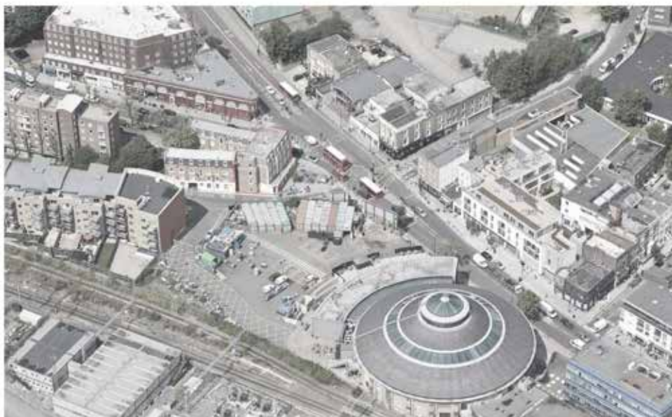
AERIAL VIEW OF EXISTING SITE
