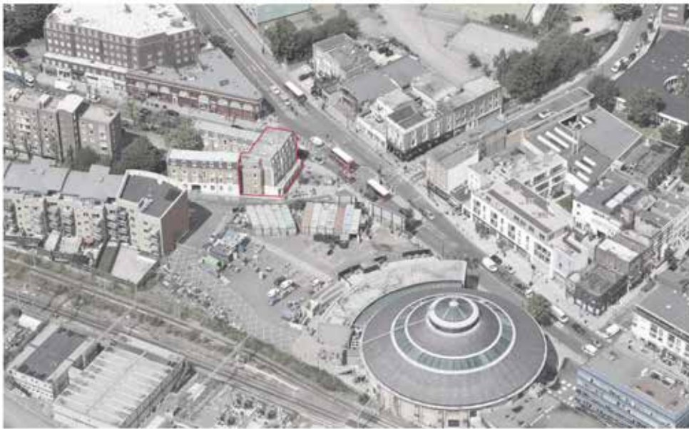
AERIAL VIEW OF EXISTING SITE
