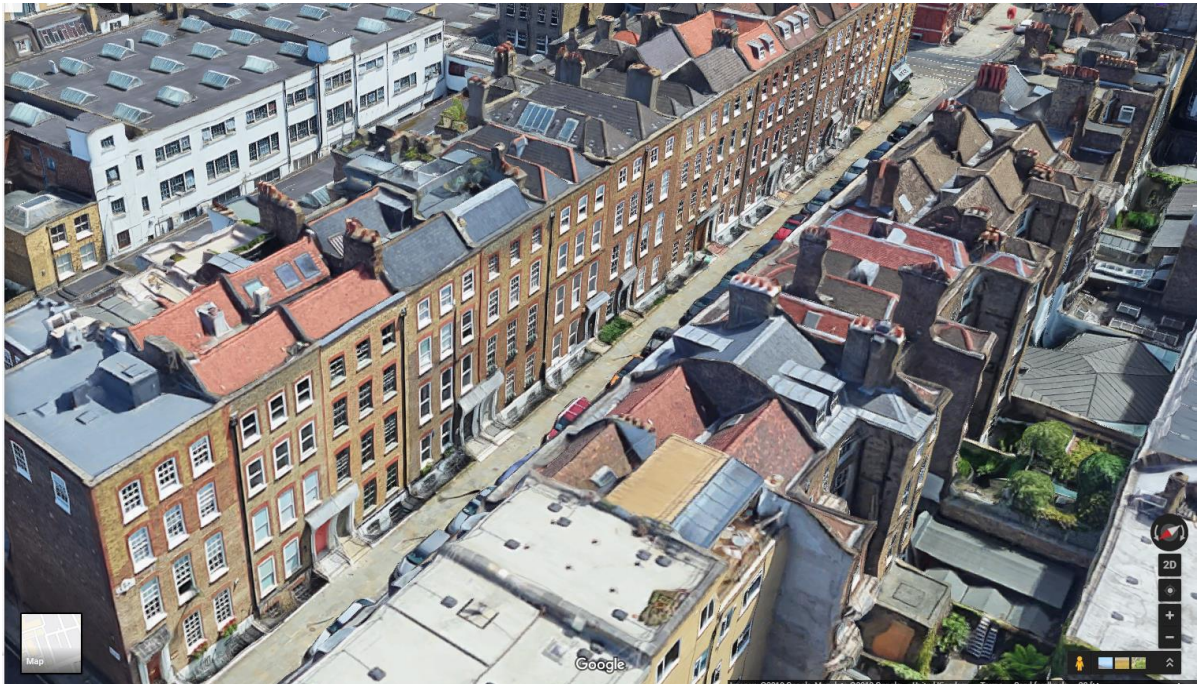
Fig.04: Existing building: 15 Great James St, showing streetscape looking towards Theobalds Rd.
