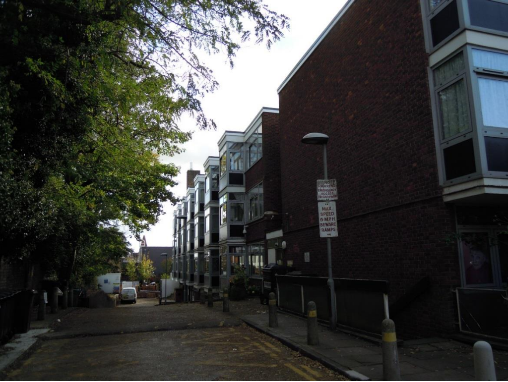
3) View of chimney tower along side access road from Prince Arthur Rd
