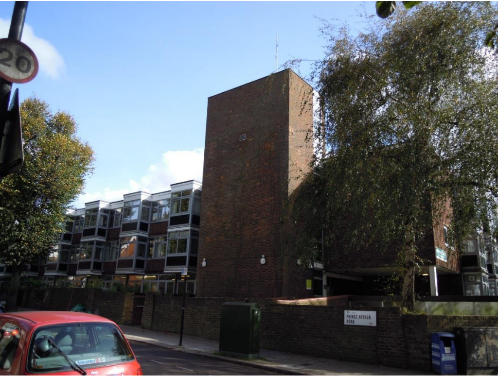
4) View of plant room tower from Prince Arthur Rd
