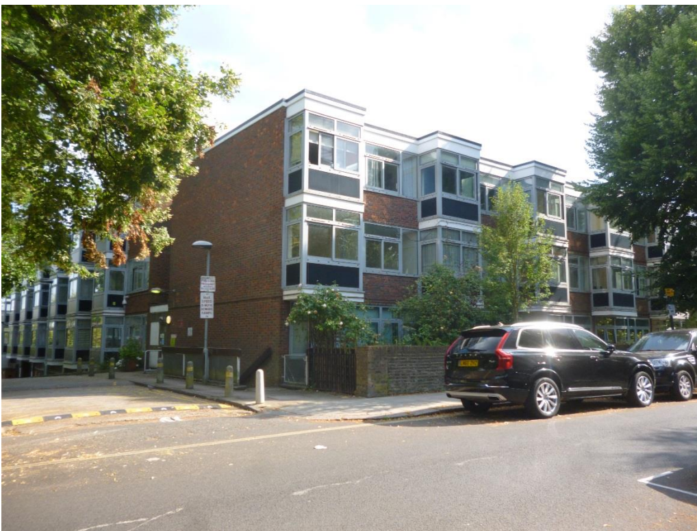
2) General view along Prince Arthur Road
