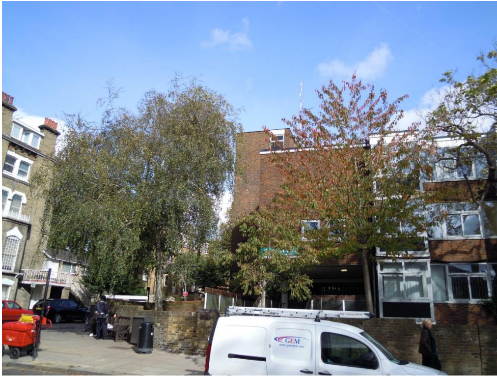
5) View of plant room tower from Fitzjohn's Avenue
