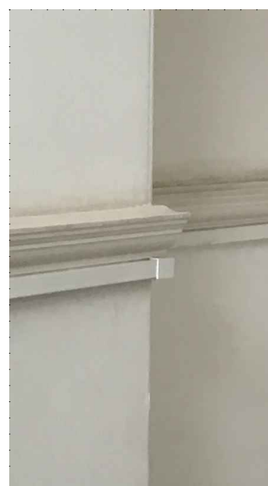
Photograph of existing dado rail moulding
