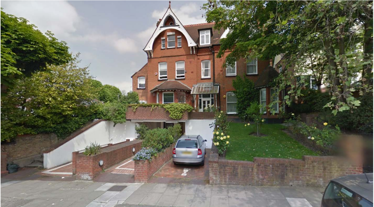
Above: Front Elevation showing character, access and vehicle hard-standing on site.
