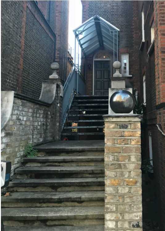
Photo of Upper Level Staircase
