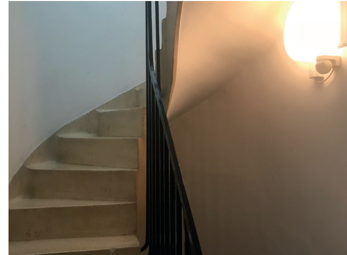
Figure 5.32 Second floor back stair
