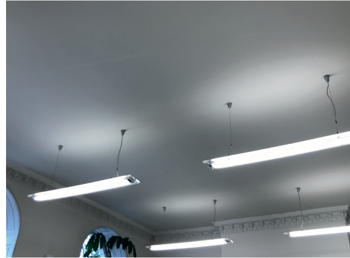
Figure 5.8 Ground floor Reception room
