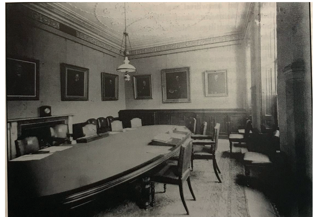
Figure 3.3 c.1883 decorative ceiling shown now lost
