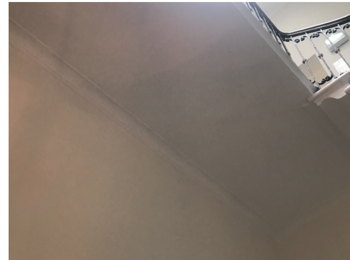
Figure 5.18 Underside of the cantilever staircase
