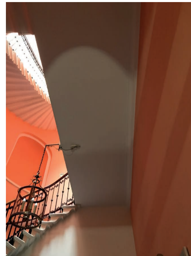
Figure 5.11 Ground floor looking up to one of the cantilever staircases
