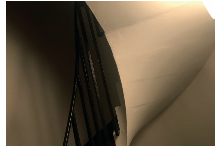
Figure 5.26 Back stair at first floor level
