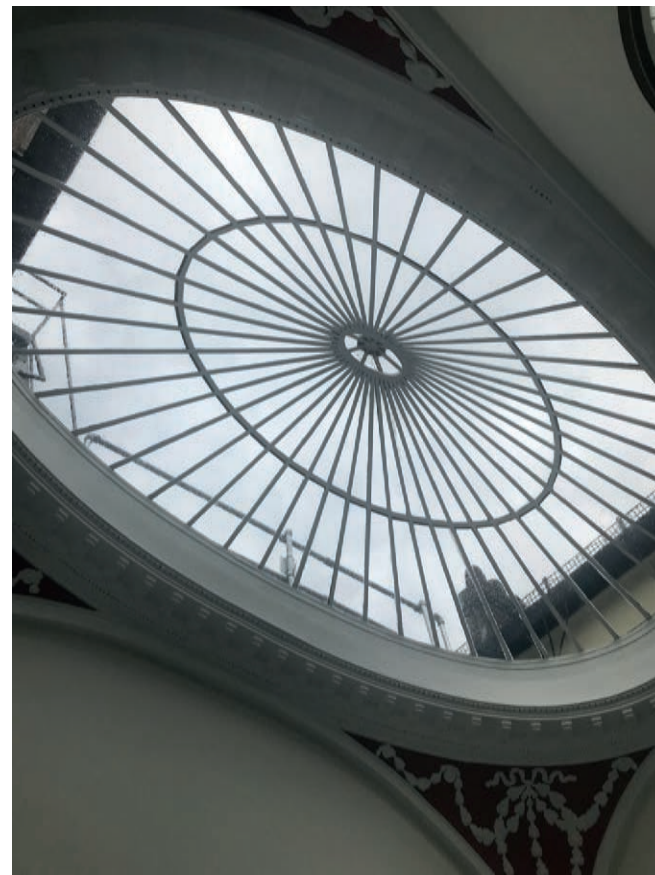
Figure 5.31 Second floor grand staircase glass roof lantern
