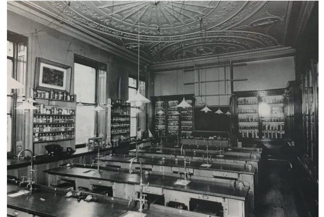
Figure 3.6 1931 first floor room fitted as a laboratory
