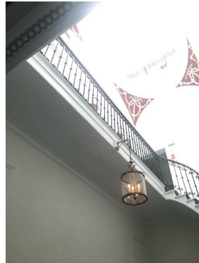
Figure 5.25 Grand staircase from first floor, looking up towards glass lantern
