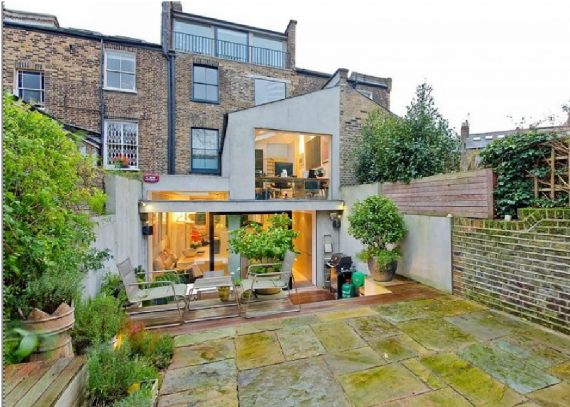
2. View of the rear elevation
