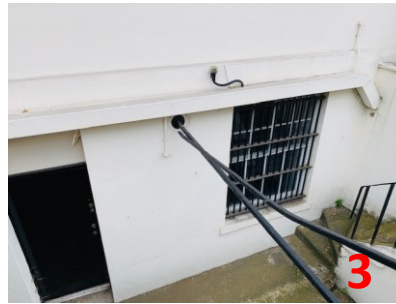
Front lightwell 9 MS - previously installed service light removed
