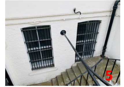
Front lightwell 11 MS - previously installed service light removed
