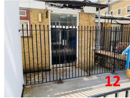
Railings to rear of 10 MS – 1850mm high
