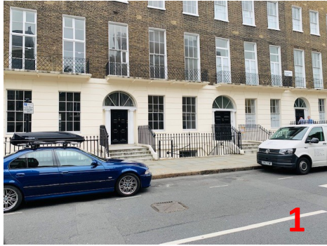
Front elevation 8-11 MS - all external lights confirmed removed
