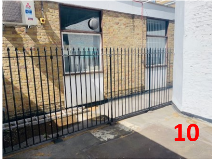
Railings to rear of 8 MS – 1850mm high
