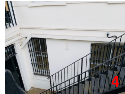
Front lightwell 10 MS - previously installed service light removed
