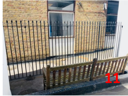
Railings to rear of 9 MS – 1850mm high
