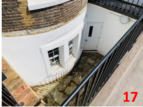
Lightwell to rear of 10 MS reinstated
