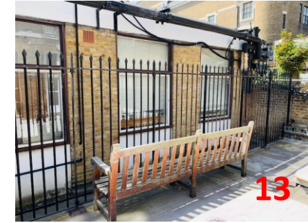
Railings to rear of 11 MS – 1850mm high
