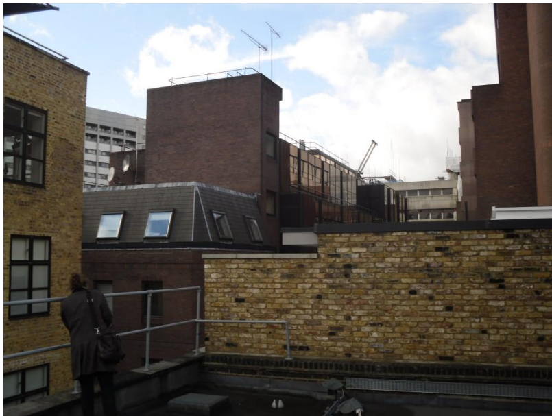
View looking back to No. 18 Stukeley Street from roof
