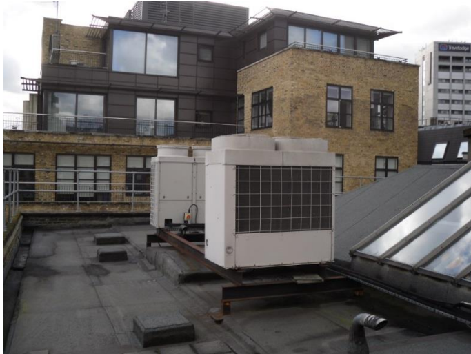
Existing roof of host building
