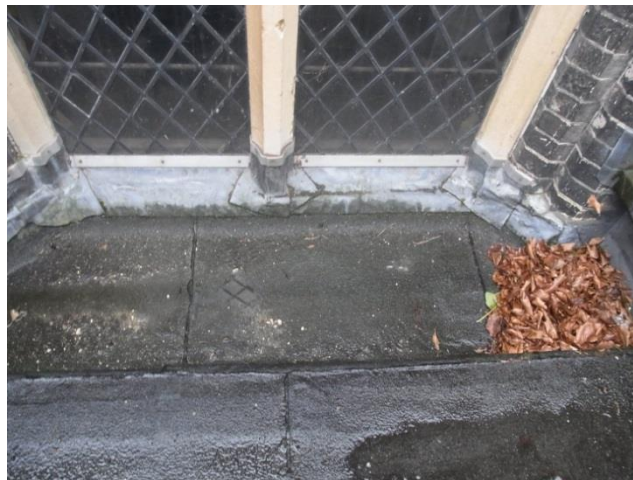
Link roof, window sill and catchpit
