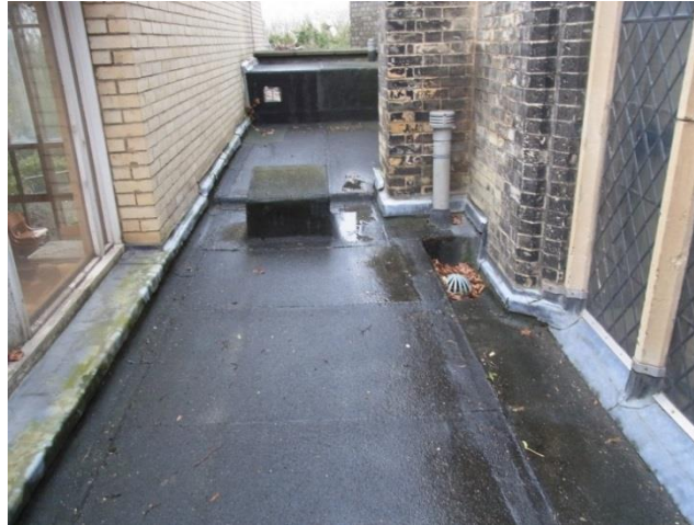
Link roof, view towards the back (East)
