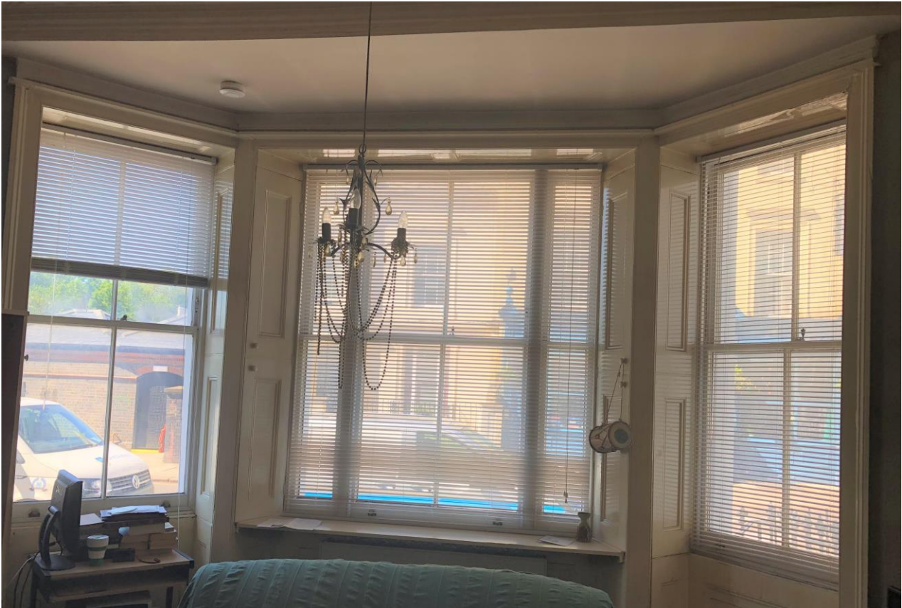
Figure 4: Internal view of windows at ground floor level – lounge (Flat A)
