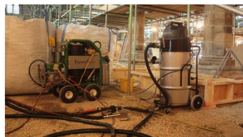
Photo Lower Right: ThermaTech and ThermaVac systems connected together for use with internal work. The recovery head is pictured in the foreground.
