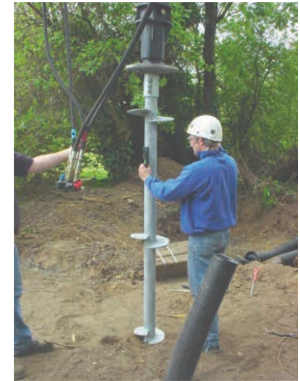
Image of Screw pile installation
