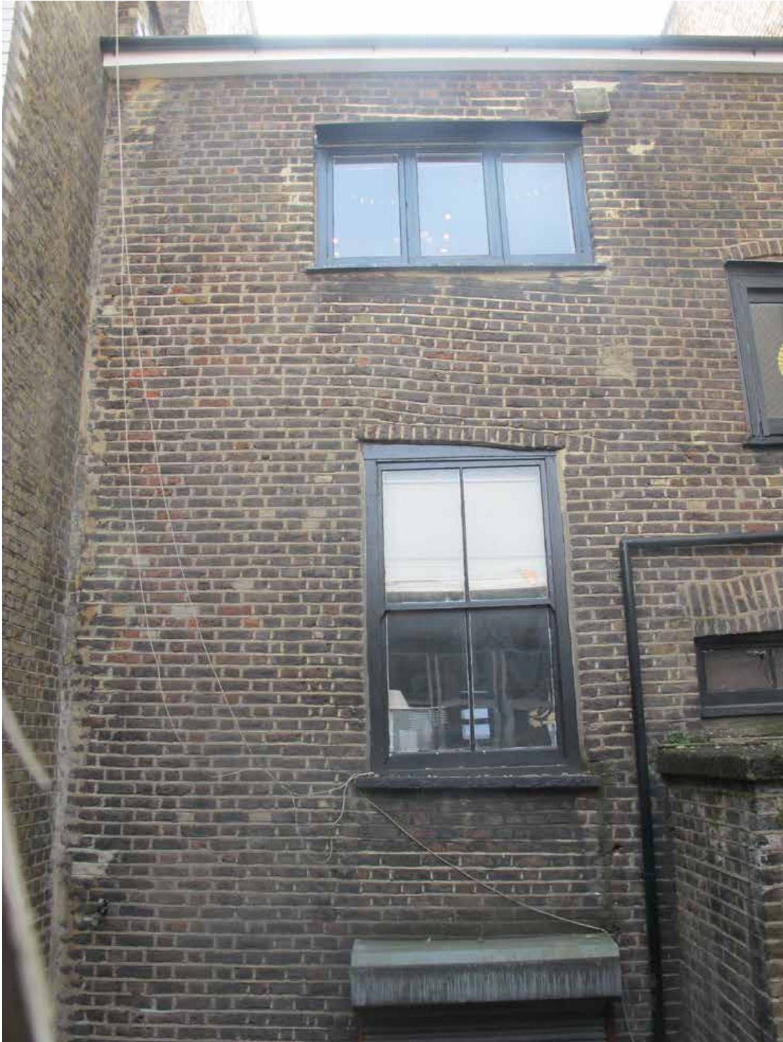
Fig. 15: View of the back elevation of No. 20 Denmark Street
