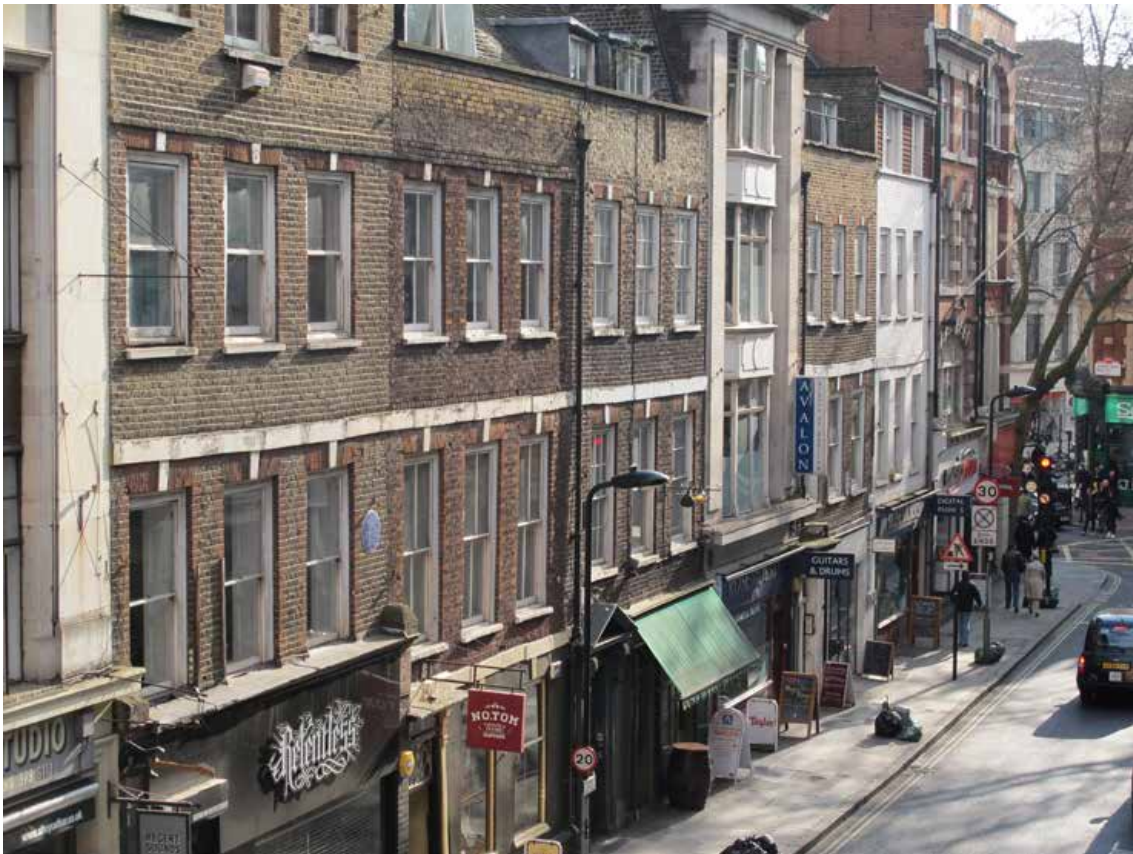
Fig. 16: General View of Denmark Street, looking west
