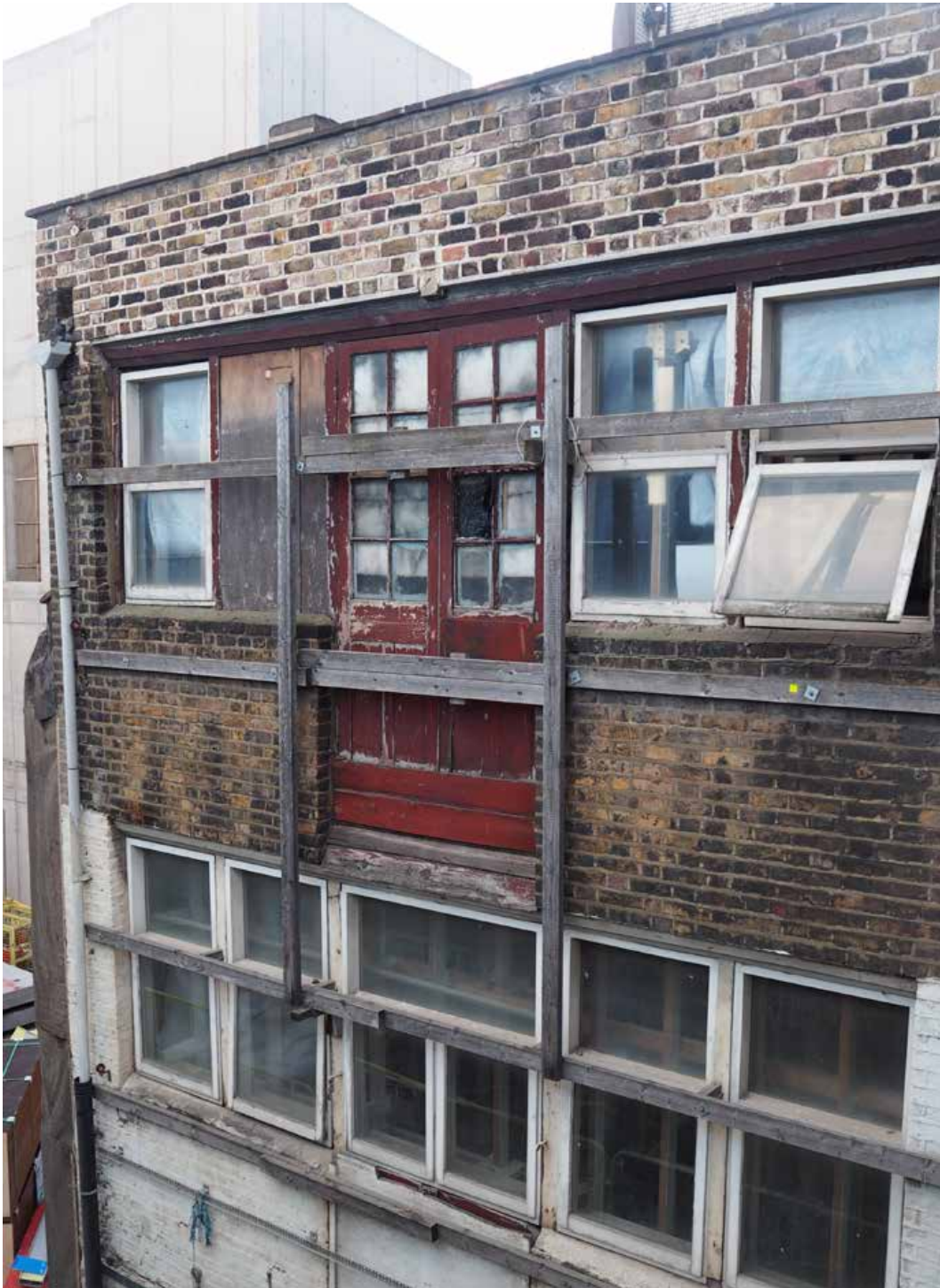
Fig. 10: The north elevation of no.16 Denmark Place
