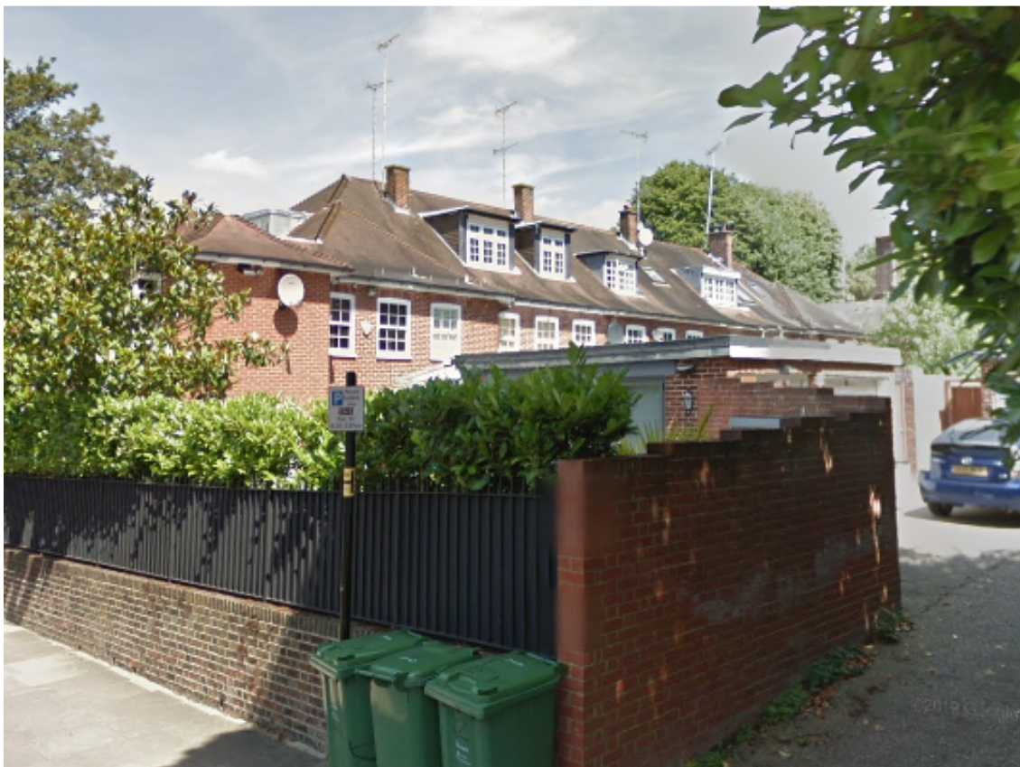
4. Rear view of terrace from no. 22
