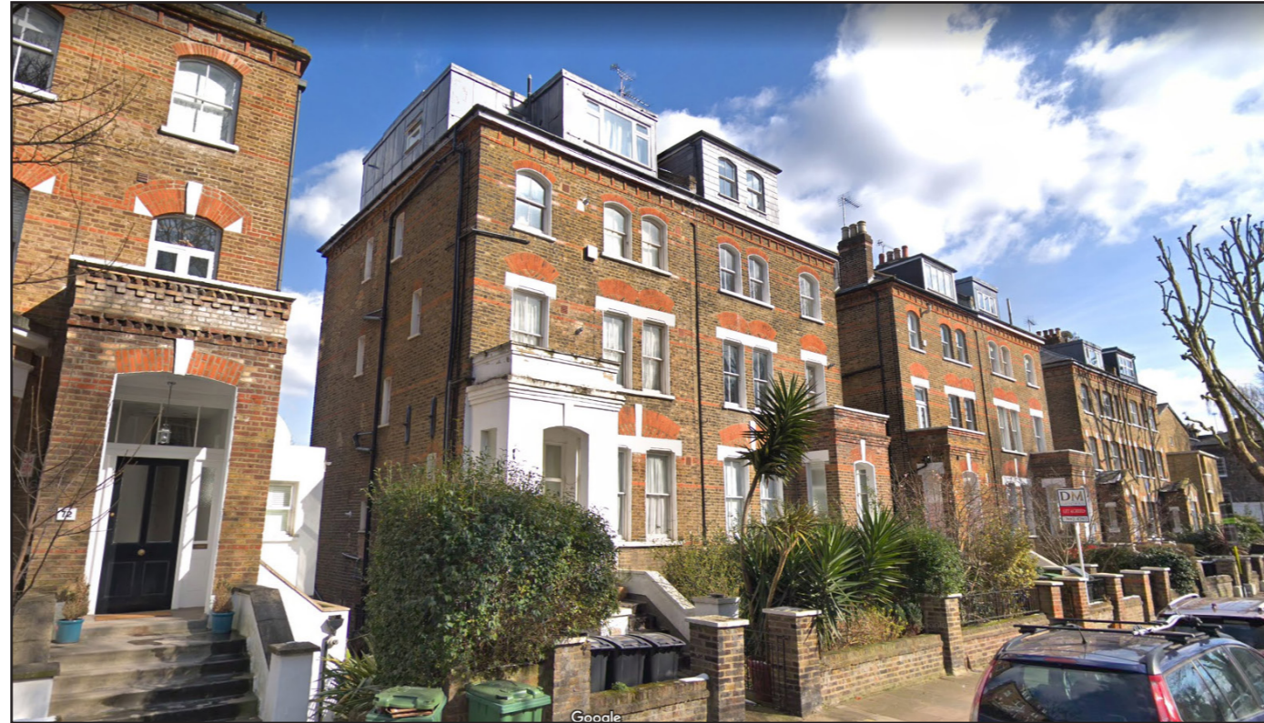
View South along Parkhill Road - Existing side and front dormers
