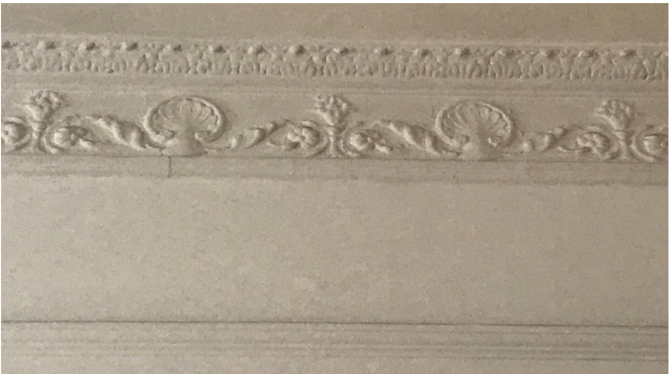
Ground Floor Front Reception Room – ceiling cornice detail
