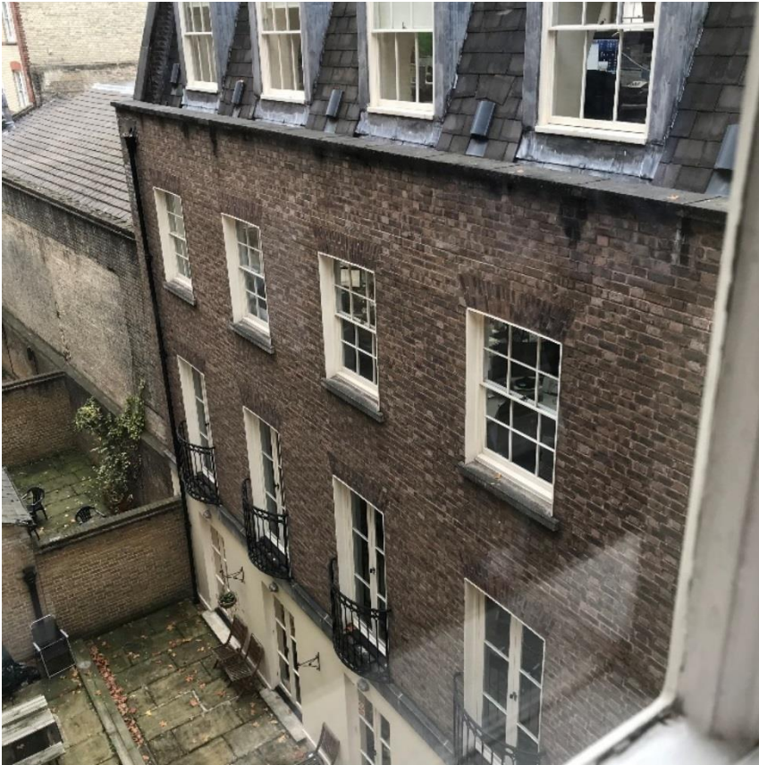
Façade of rear building
