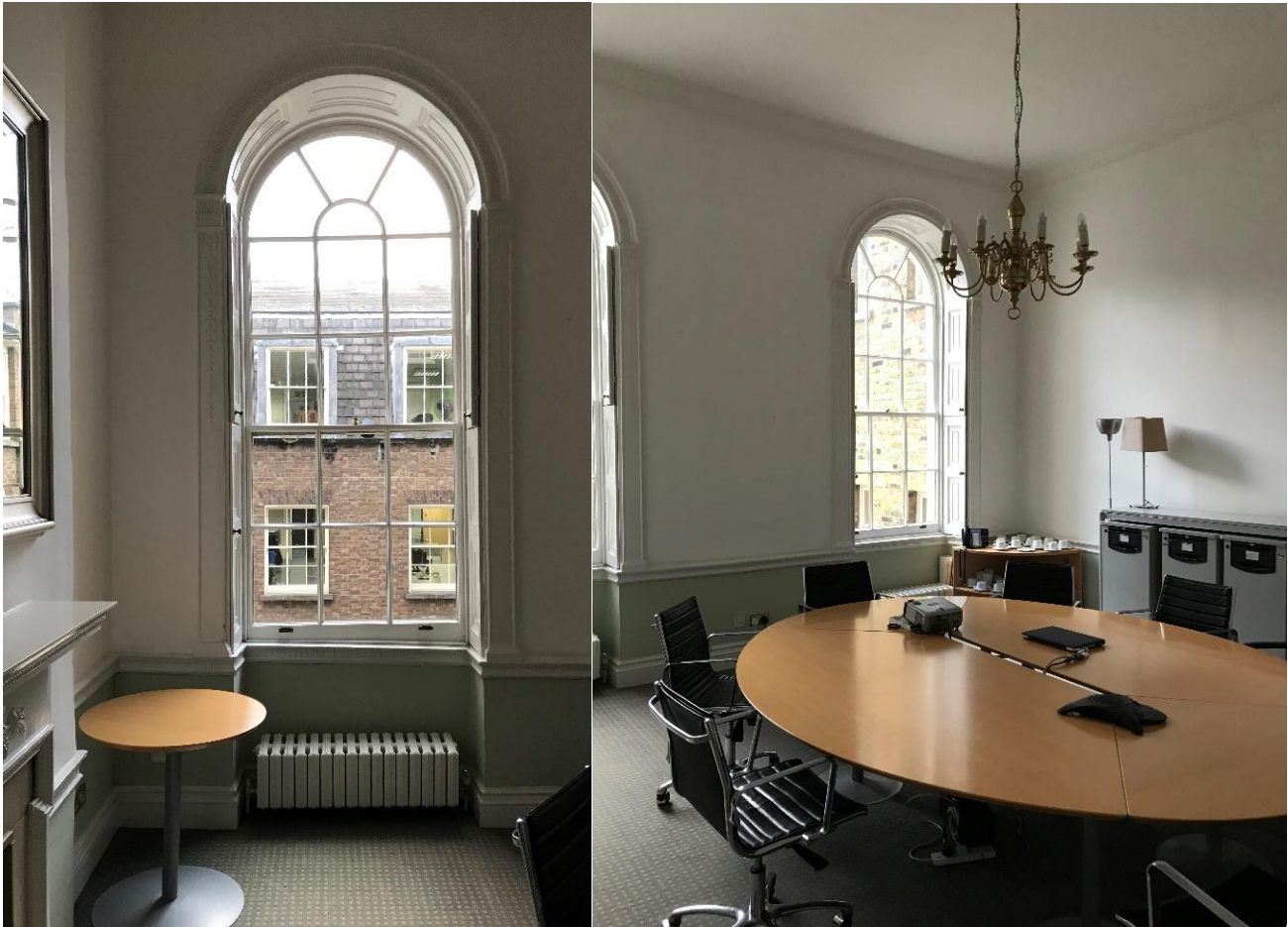
First Floor Rear Room (Grosvenor Room) – window / general view
