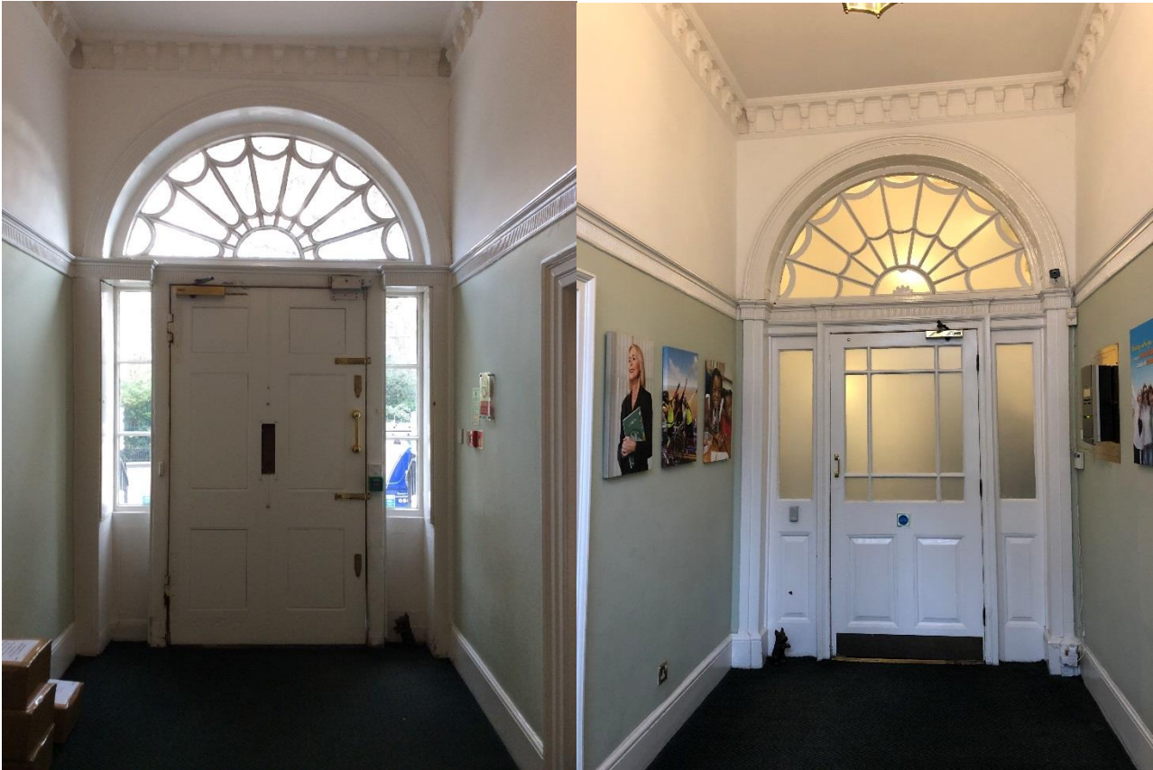
Ground Floor Vestibule – Entrance door / interior door to stairwell
