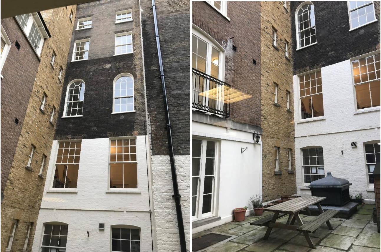
Rear Façade of Townhouse / Rear elevation(s) at Lower Ground level
