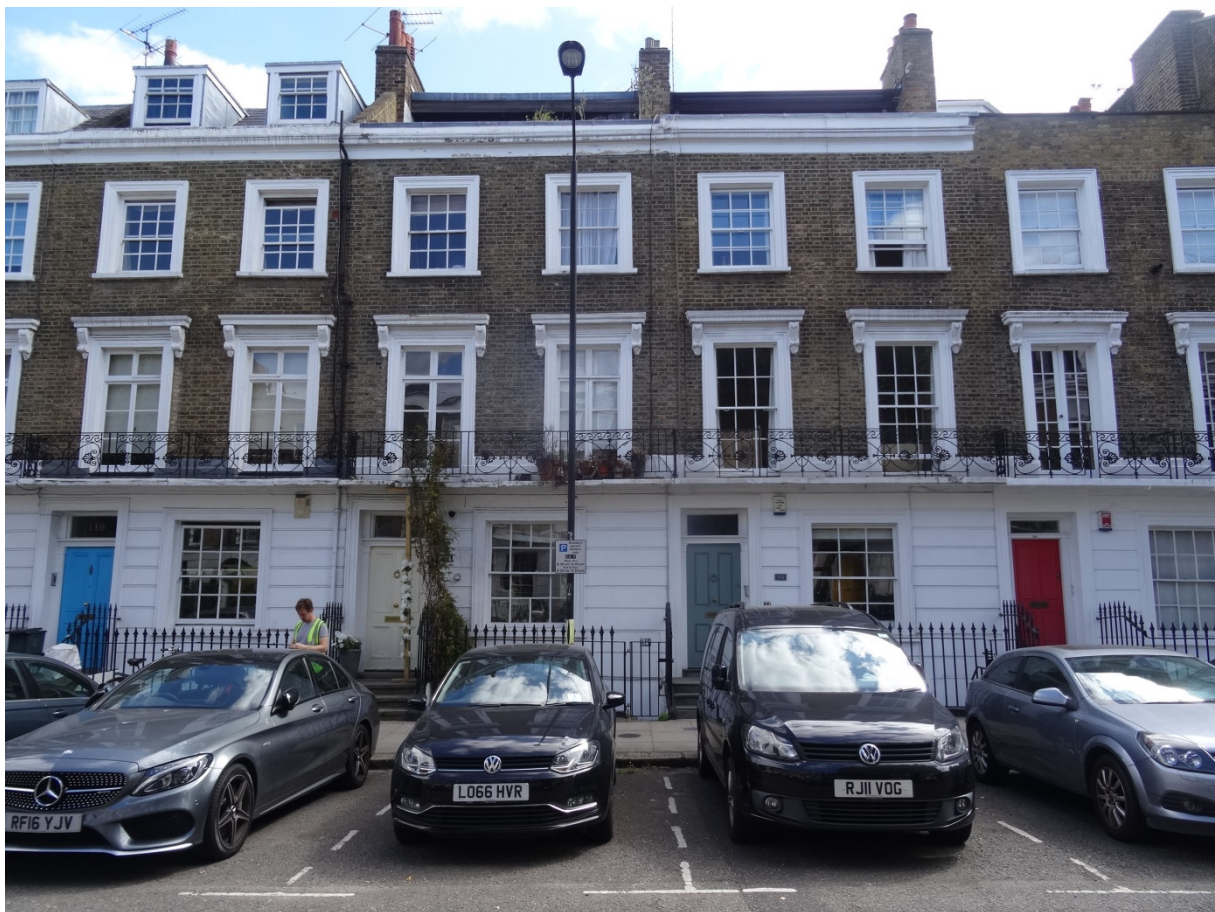
General view of the North side of Albert Street. No.114 has a prop to the balcony slab
