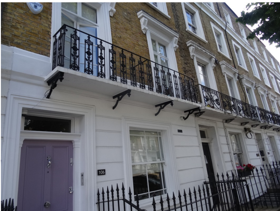
Nos. 106 to 102, with rather conspicuous iron brackets, clearly not original
