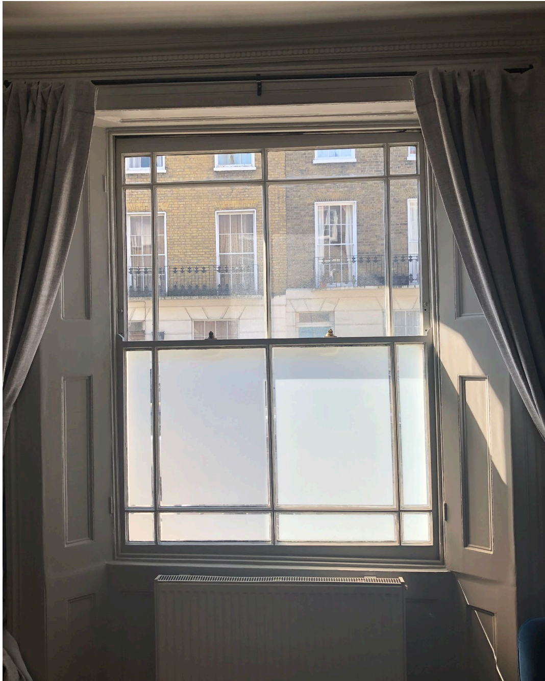
Figure 7: Internal view of window at ground floor lounge (Flat A)
