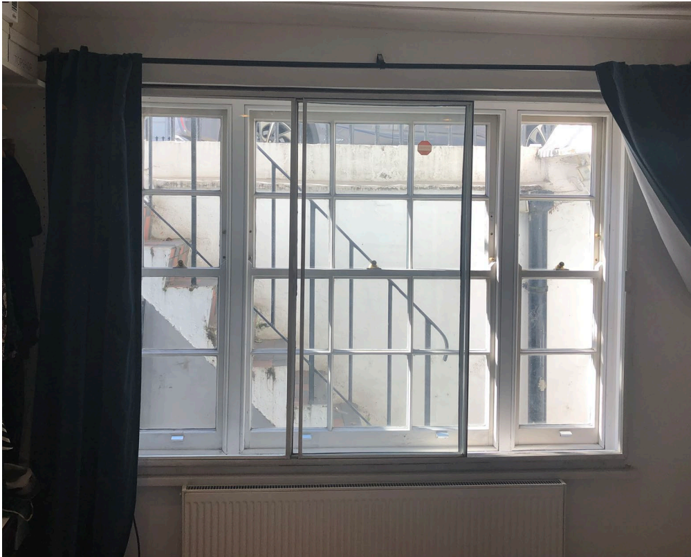
Figure 6: Internal view of window at basement bedroom (Flat A)
