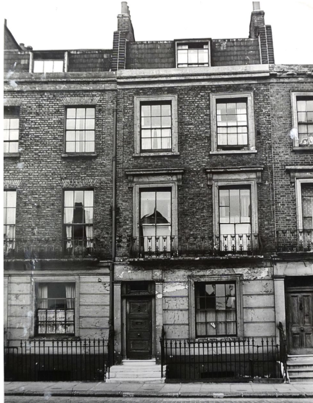
Figure 4: Photograph of 62 Delancey Street, 1958, Copyright: Camden Local Studies and Archives Centre.
