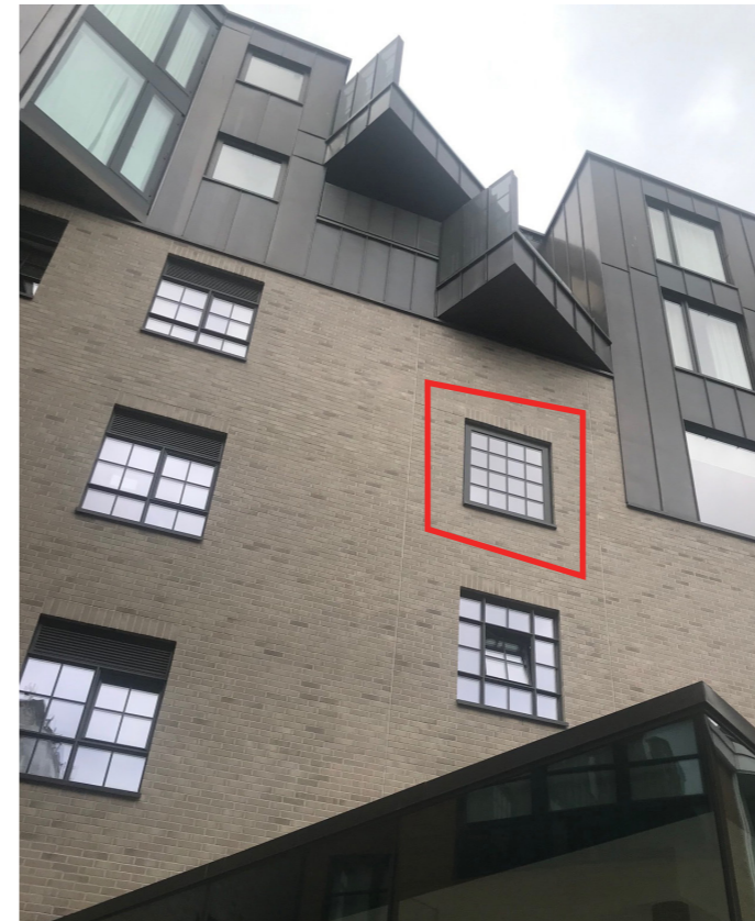
Bespoke Aluminium 'Crittall' AOV matching adjacent operable windows
