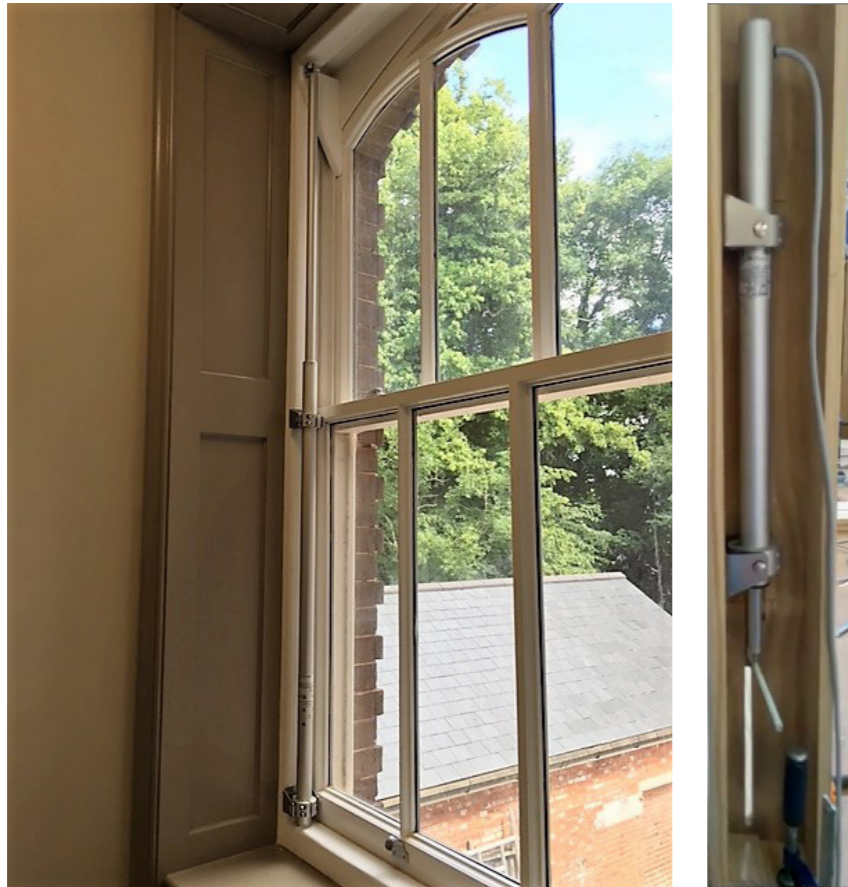
'Dummy timber sash window' with internal actuator
