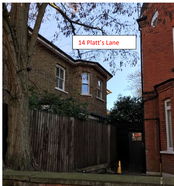
Photograph 4 - Side Elevation at No 14
