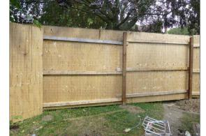
Hoarding to Site Boundary 2.4 m high Timber hoarding fixed to timber posts set at 2.0-3.0 m centres (See Photograph). Where applicable post holes for the timber hoarding will be hand dug using hand held tools and avoiding severance of significant roots of adjacent trees.
