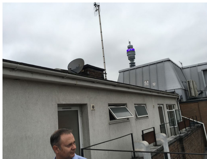
Existing fourth floor roof extension from the rear
