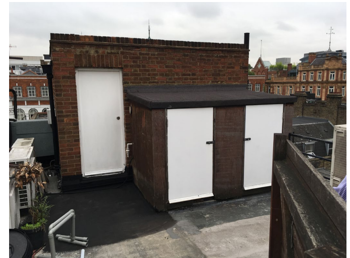
Rooftop stairwell to rear of Kirkman House
