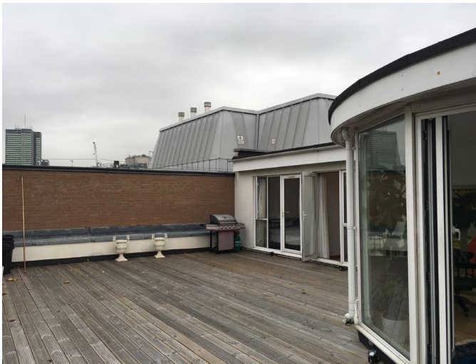
Existing fourth floor roof extension
