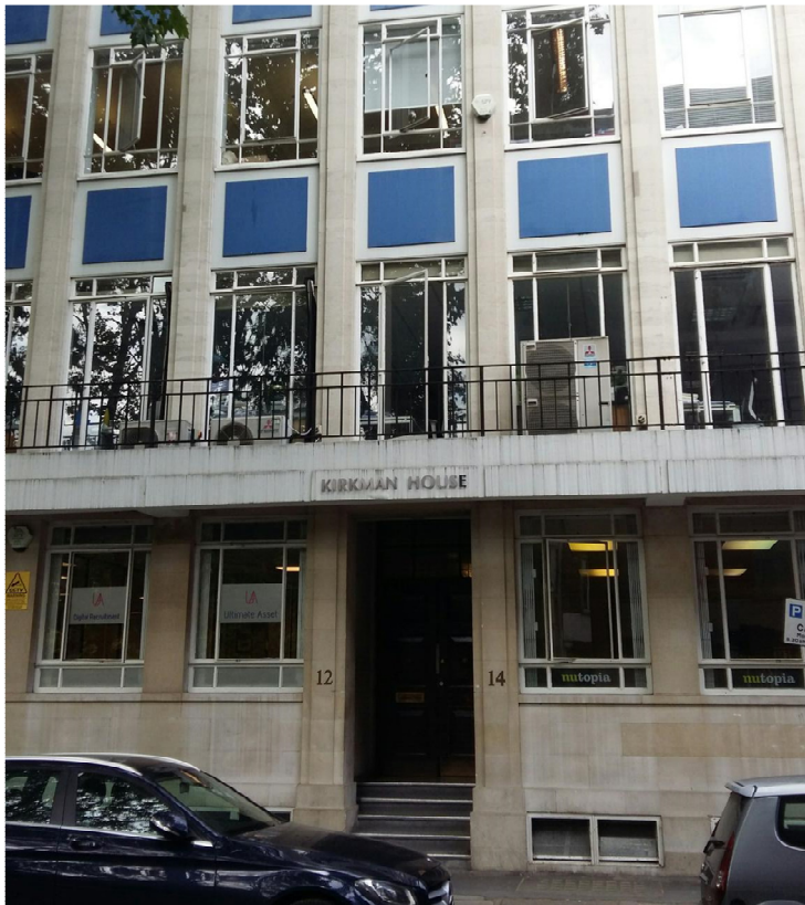
Figure 2: Photograph of existing building from Whitfield Street (source: Planning Potential)
