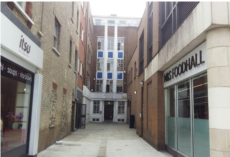
Figure 3: Photograph of existing building from Tottenham Court Road, looking down Kirkman Place (source: Planning Potential)
