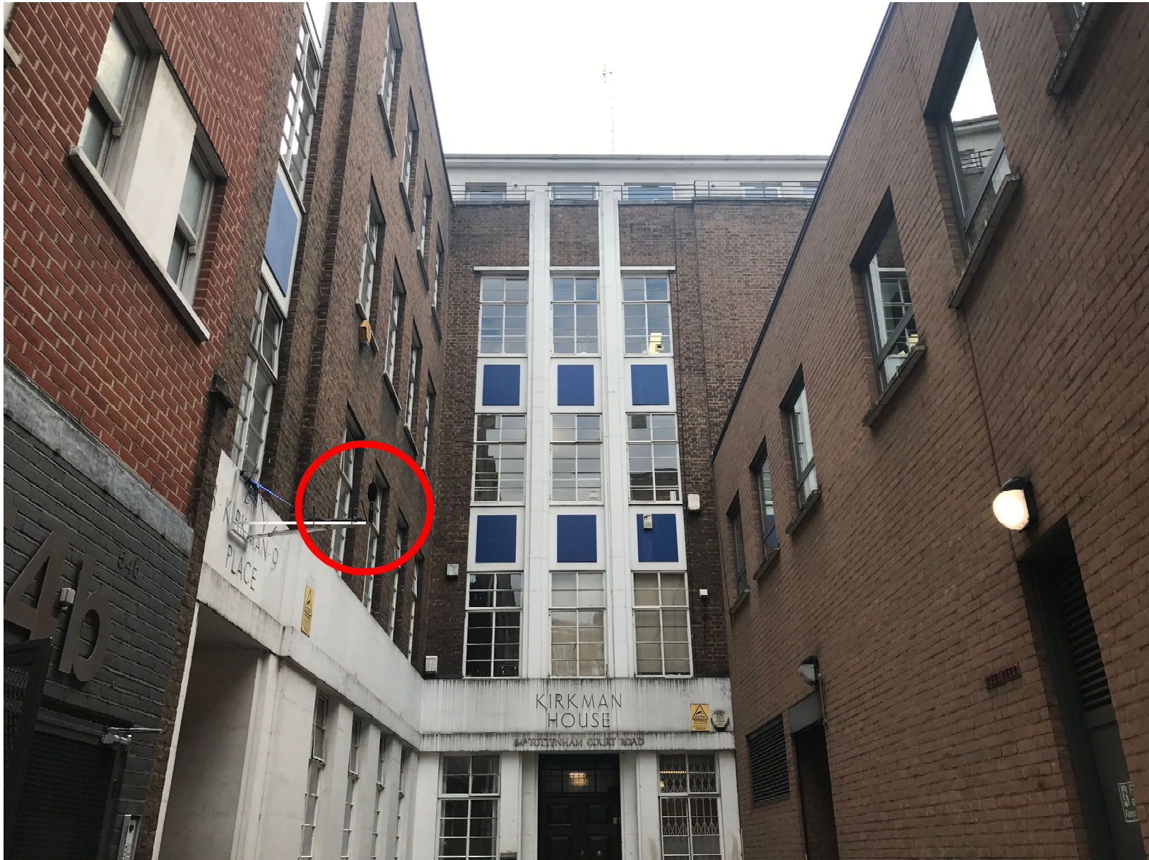
Kirkman House, 12 - 14 Whitfield Street, W1T Photo Showing Measurement Position 1 Project 9326
